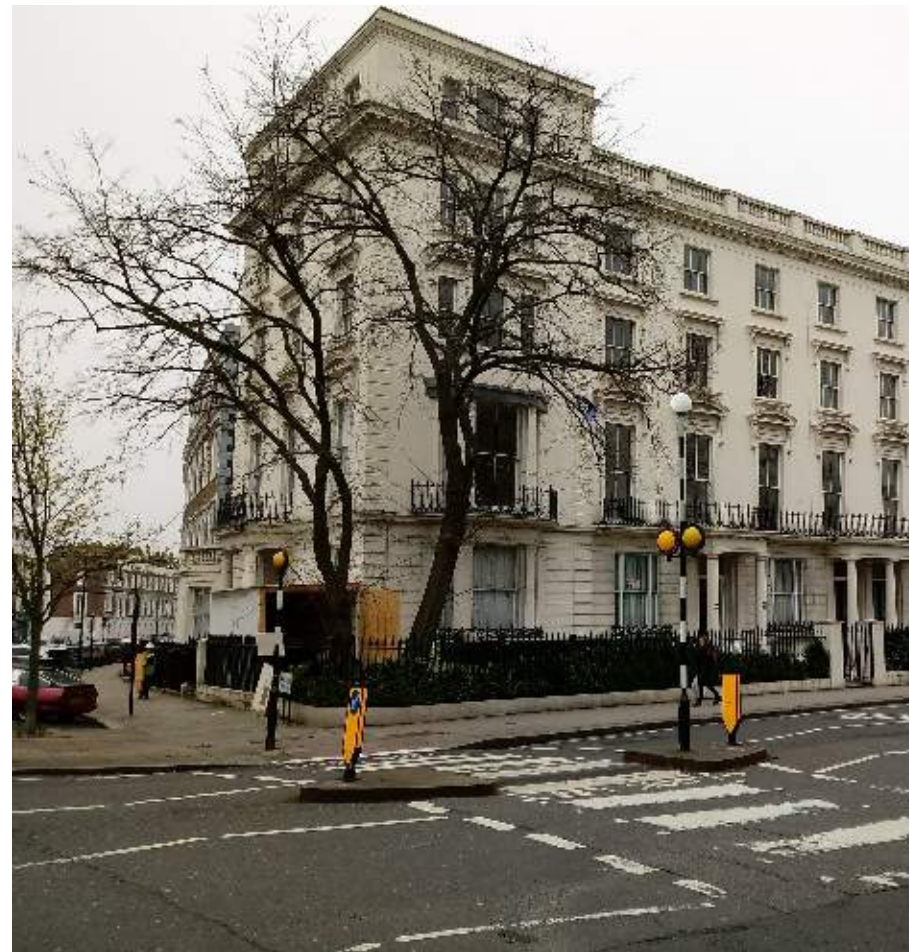
Image 07 Existing Building, street view
