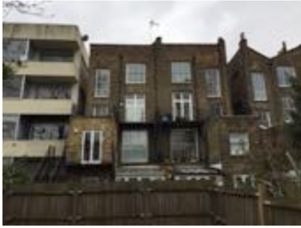
View of rear elevation of no. 8 & 9 Cliff Road.
