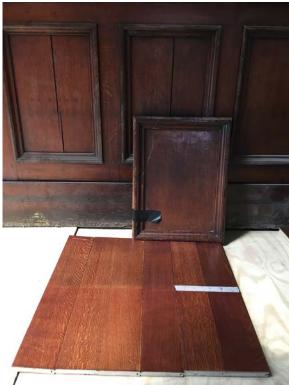
1. Photograph of sample of proposed timber flooring against existing timber wall panelling
