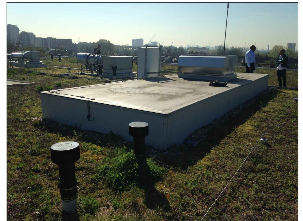
3 EXISTING LIFT OVERRUN
