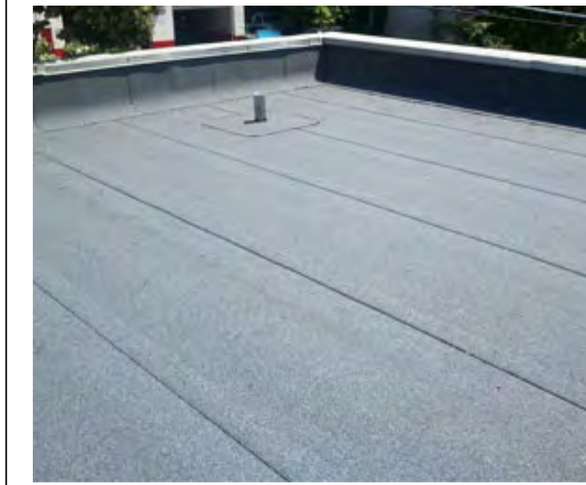
TYPE 1 - Bituminous Membrane
