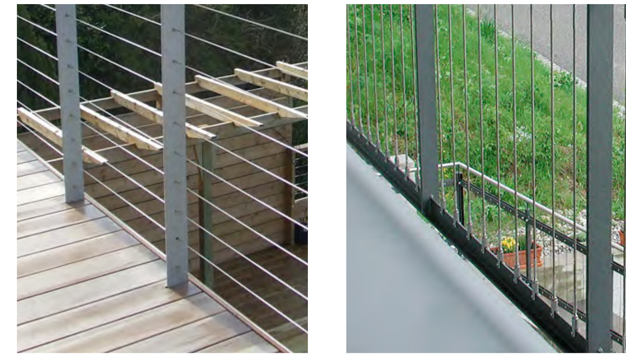
Wire guarding within perimeter wall (Vertical & Horizontal) Jakob wire rope system
