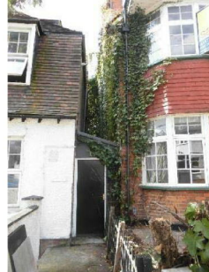
Photograph 4 – Rear boundary view with No.2 Kingscroft Road
