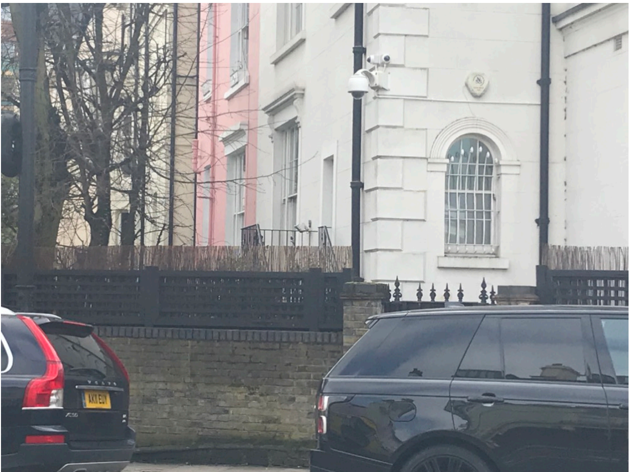
Small section of the existing balustrade visible from Regent's Park Road
