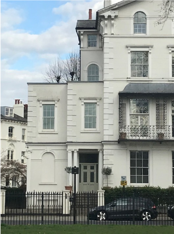
Cill to arched window at second floor not visible
