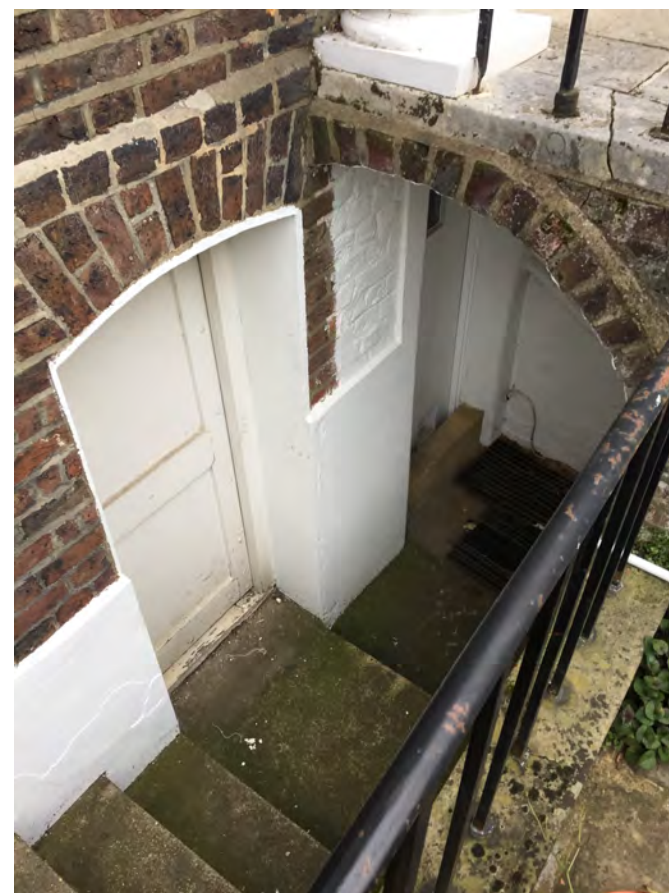
Existing basement entrance door - access to be retained
