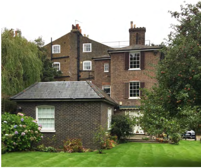
Existing rear extension - view from rear garden
