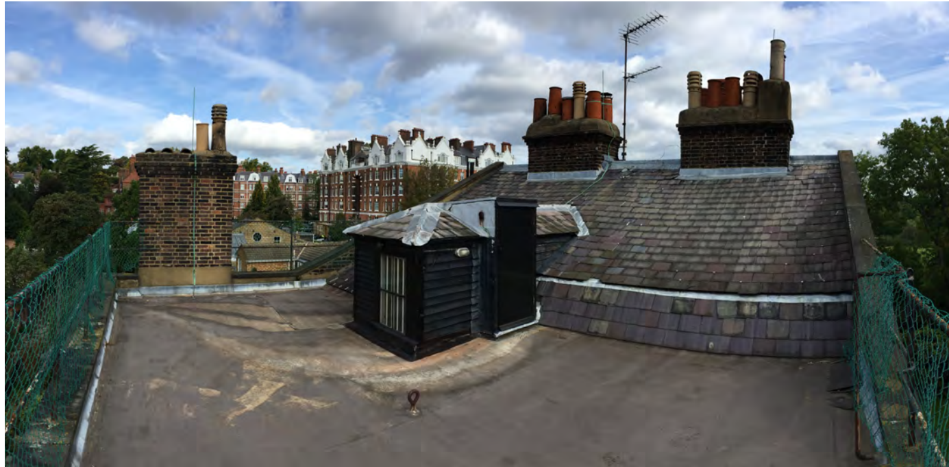
Existing roof terrace and dormer - access to be retained
