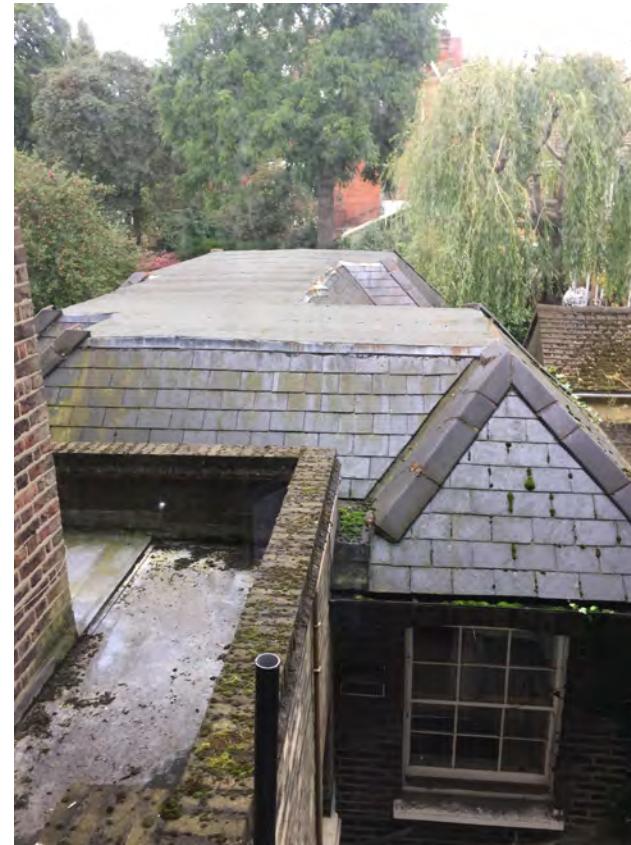
View of existing rear extension from 1st Floor half landing
