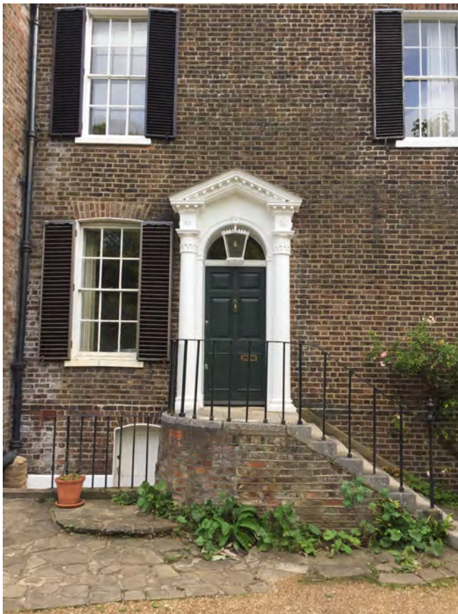
Main entrance door - access to be retained
