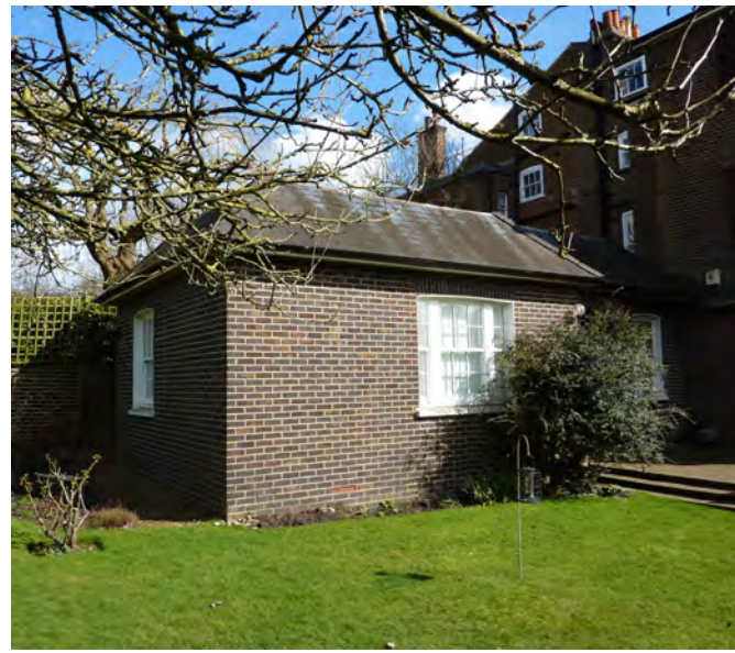
Existing rear extension - side view
