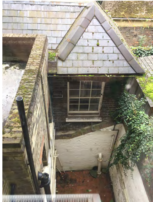
Existing side lightwell to basement
