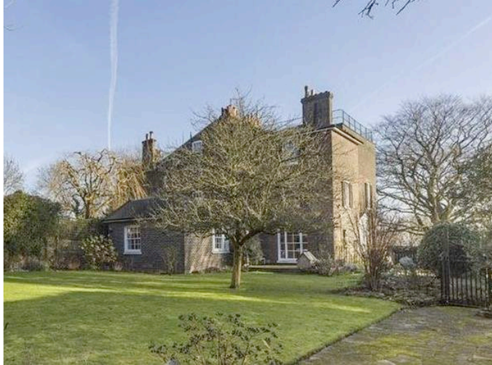
Figure 12: The single-storey rear extension of 1972
