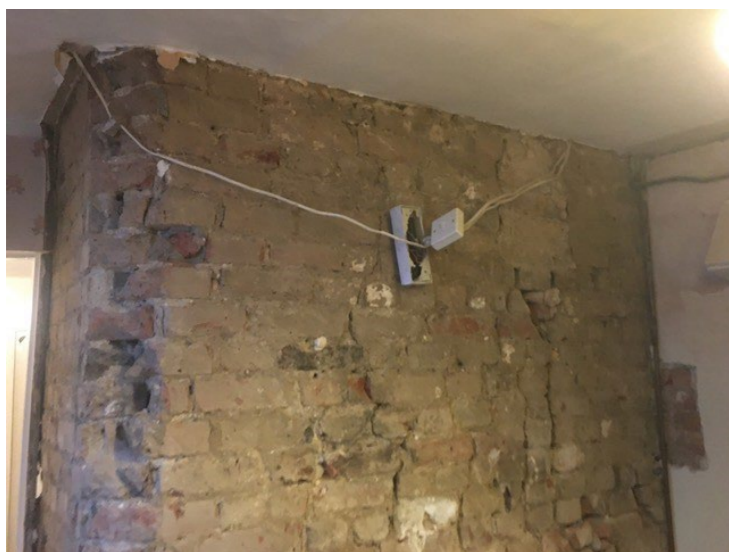
Chimney following opening up: Existing hearth at ground floor (kitchen)
