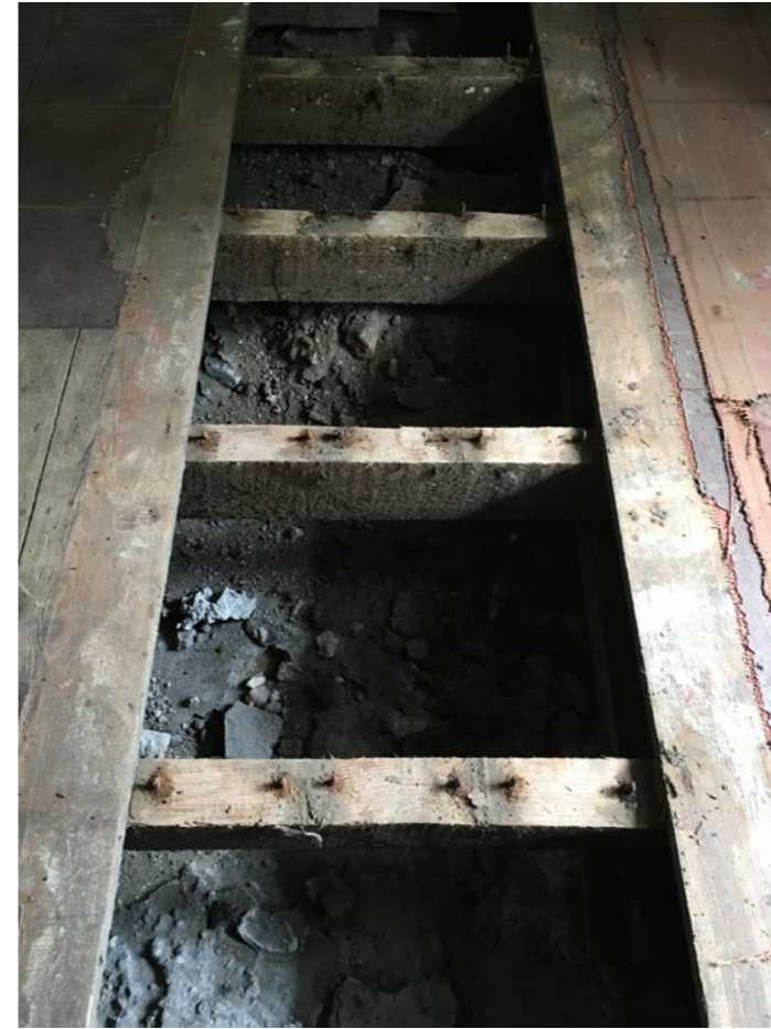
TP - 09 Flooring in body of main reception room
