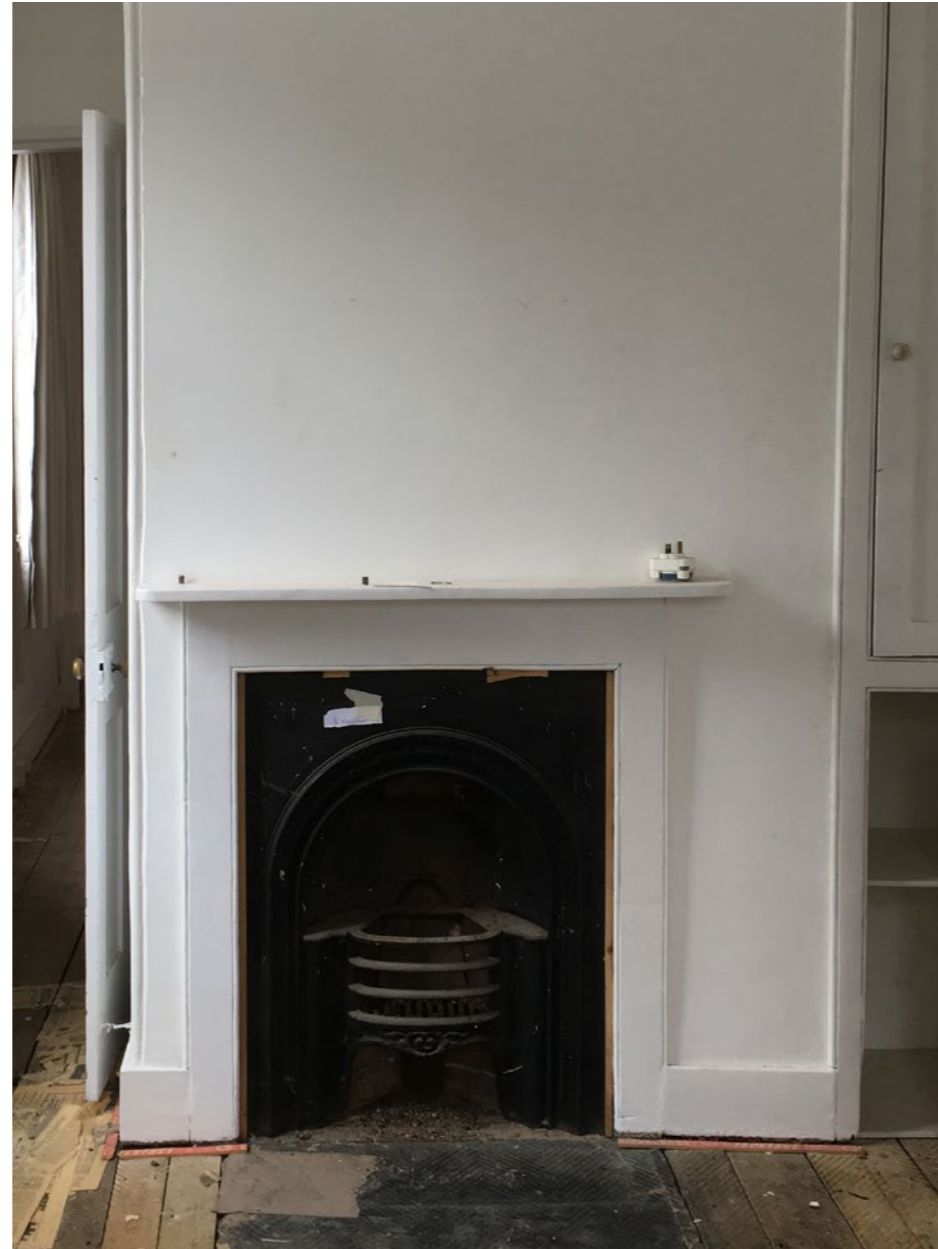
Existing fireplace in back bedroom at 1st floor (Victorian)
