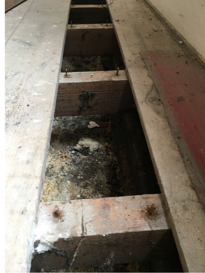
TP - 07 Flooring at ground floor adjacent to facade
