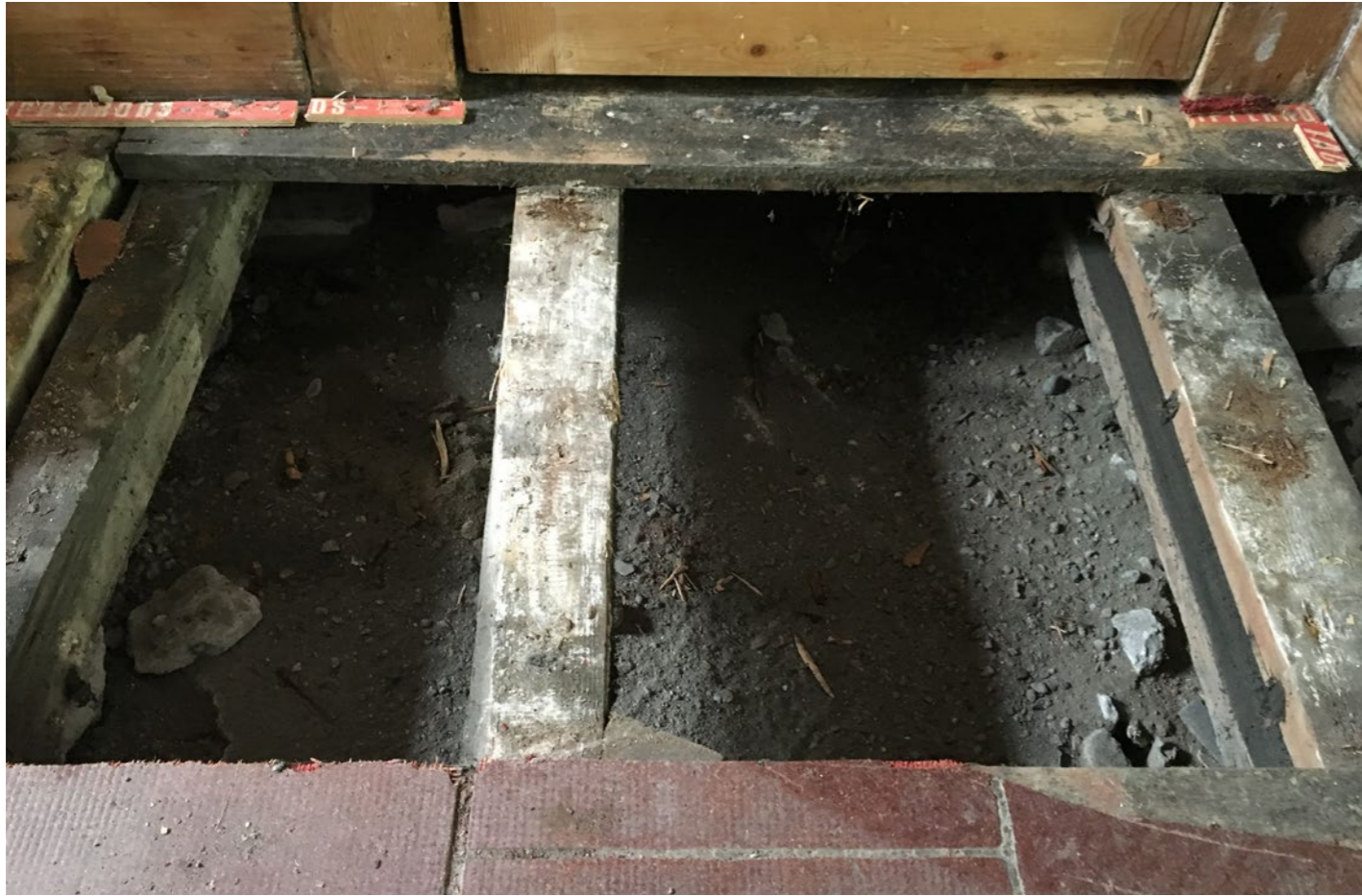
TP - 08 Flooring by hearth in main reception room
