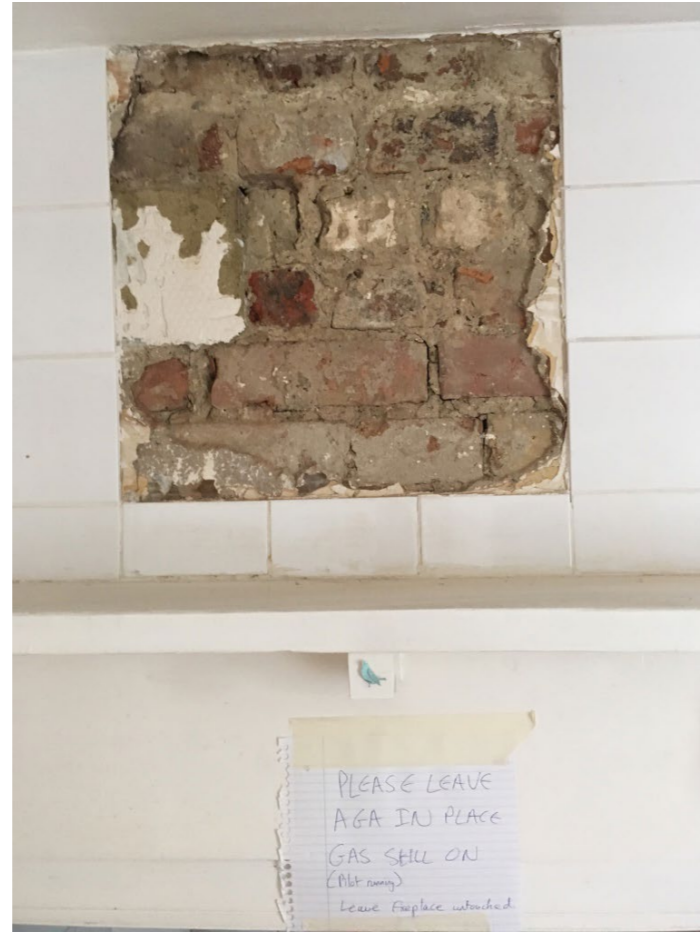
TP - 11 Finishes to existing chimney
