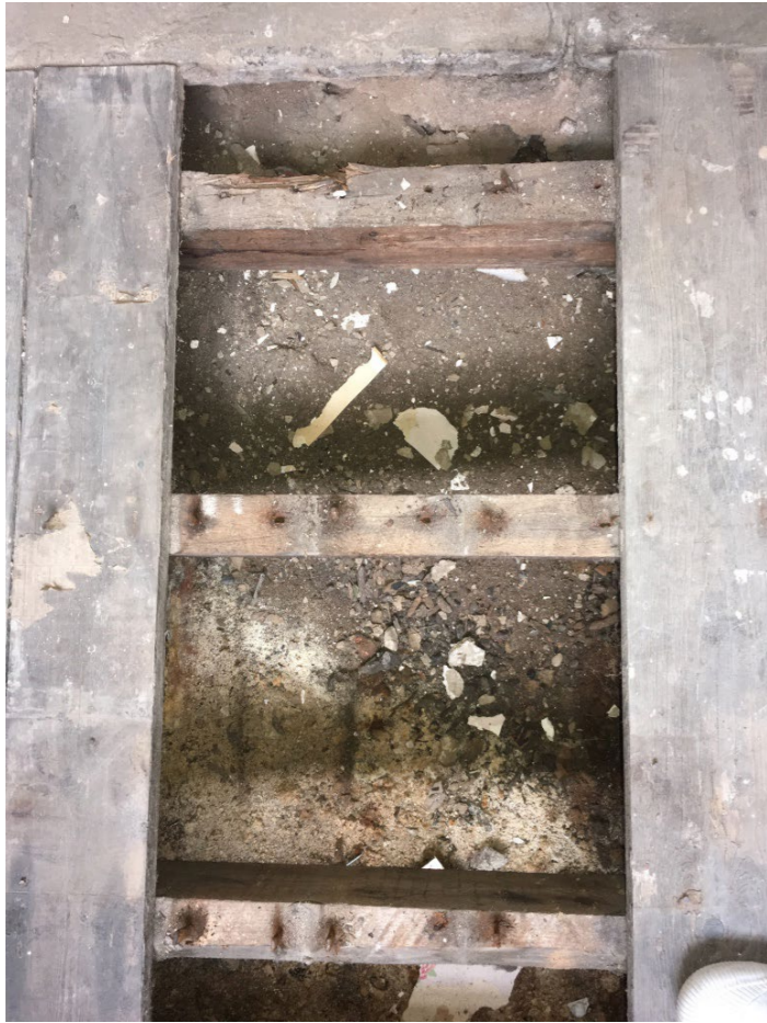
TP - 12 Floor adjacent to kitchen chimney
