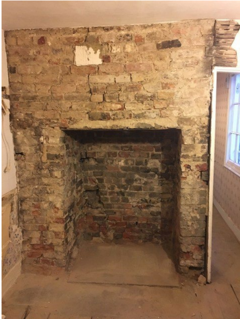
Chimney following opening up: Existing hearth at ground floor (kitchen)
