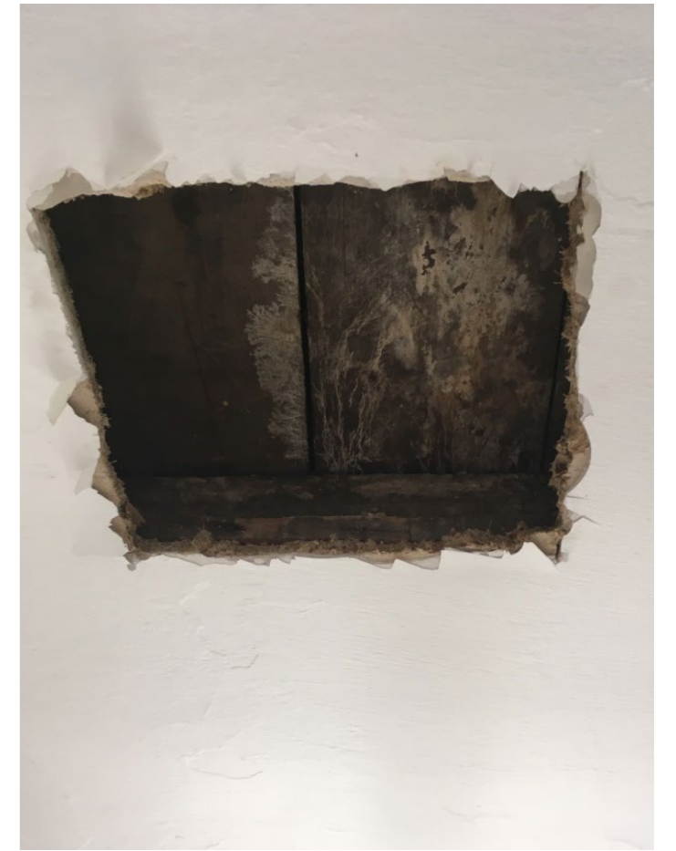
TP - 14 Footing for balcony
