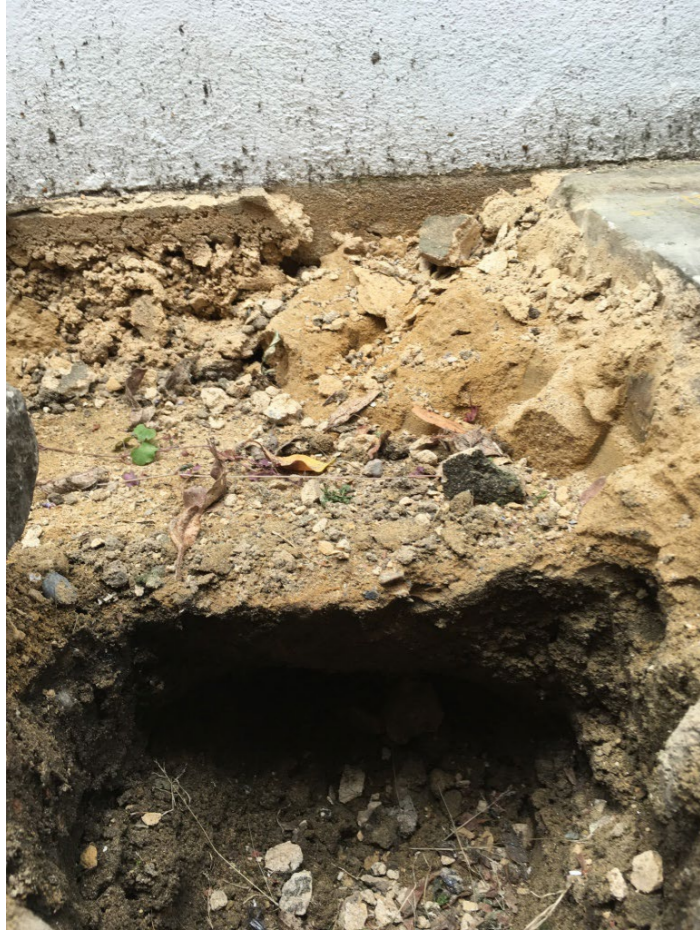
TP - 05 Exterior paving
