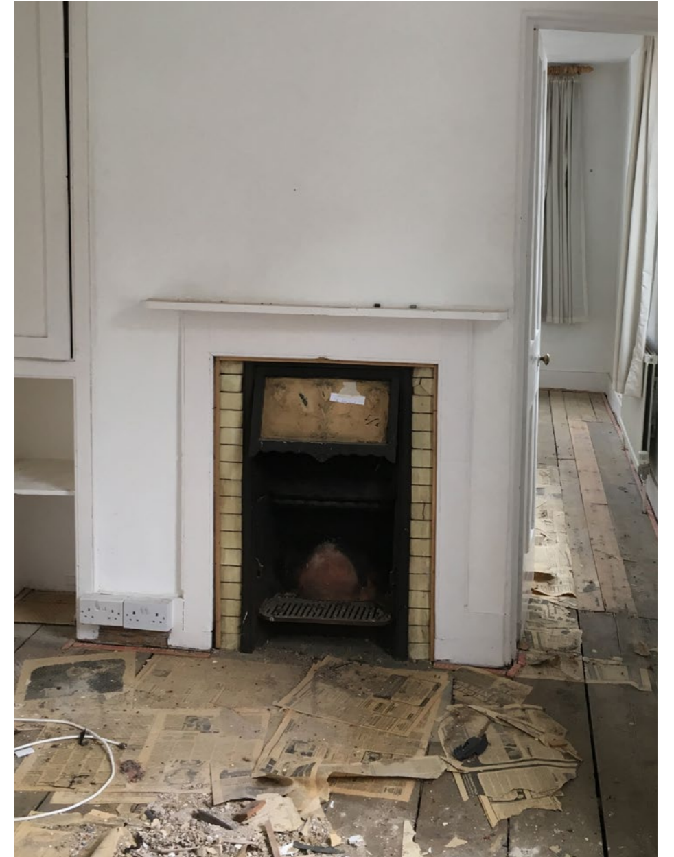
Existing fireplace in middle room at 1st floor (likely Edwardian)
