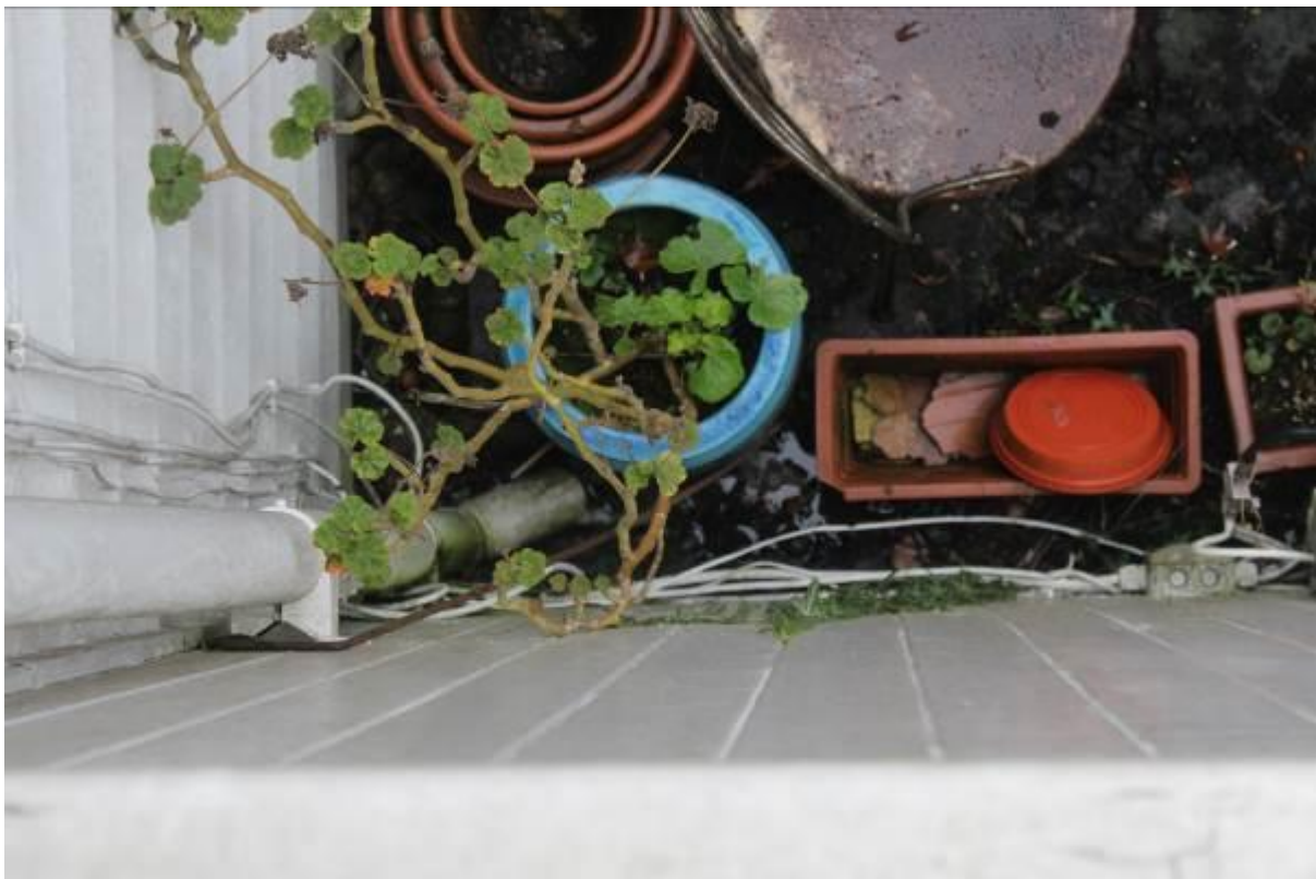
20. Rainwater build up noted in adjoining property to downpipe serving west elevation roof. Further investigation and repair/unblocking is required.
