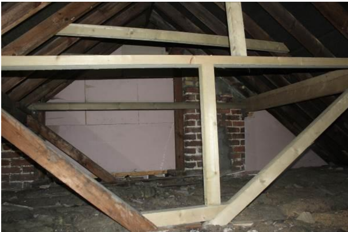
33. Additional roof supports and fireproofing of party wall to main roof space.
