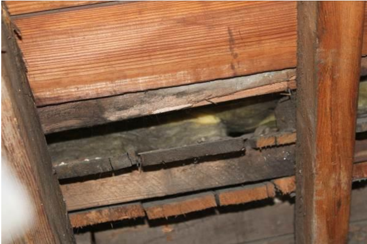
32. Evidence of some insulation in back addition roof space as viewed from the front roof space. An access hatch in this roof space is recommended.
