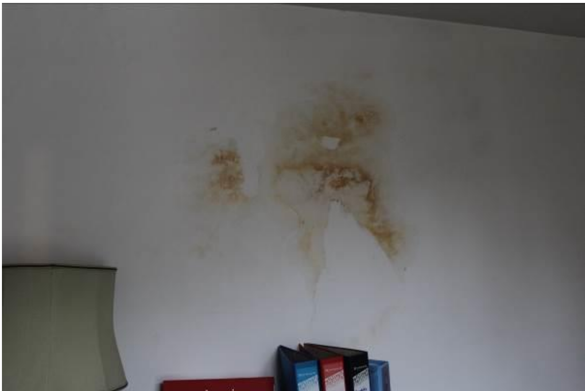
24. Plaster repairs required to first floor bedroom where water damage has occurred.
