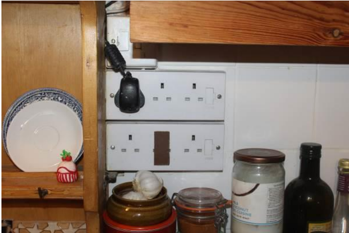
46. Poorly designed electrical socket facilities, also note one of the positions has been blanked off with tape. Further investigation or rewiring required.
