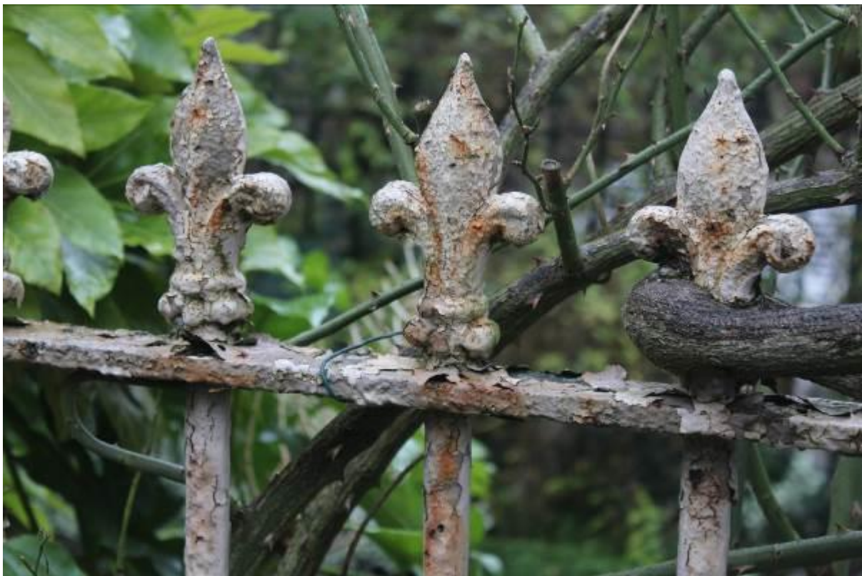
8. Redecoration required in conjunction with careful removal of corrosion to boundary railings.
