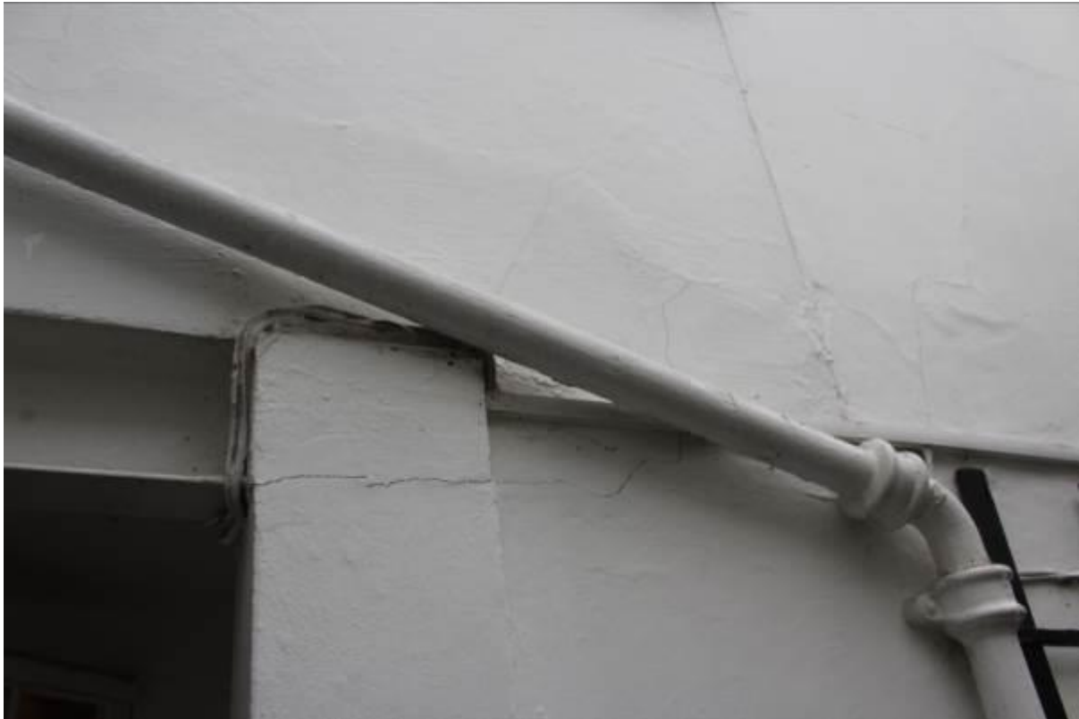
28. Some cracking observed to rear addition masonry indicating the movement is slowly ongoing.
