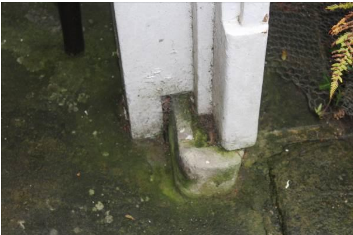
29. Front balcony support base now out of alignment and in need of re-seating.
