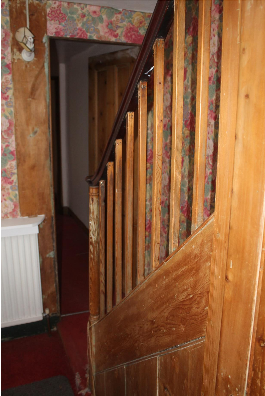
Fig.14 The lowest flight of the stair, with its turned newel and stick balusters
