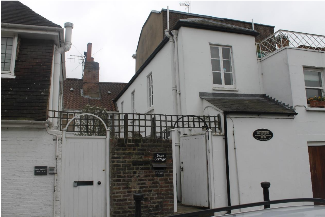
Fig.9 The rear elevation with the long rear wing
