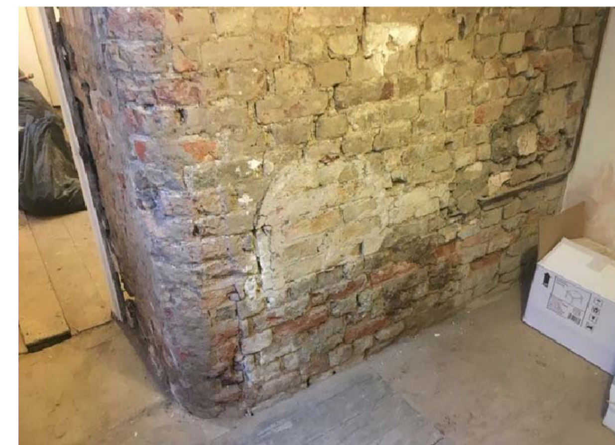
6 PHOTO OF EXISTING Elevation from sink room (lower portion)
