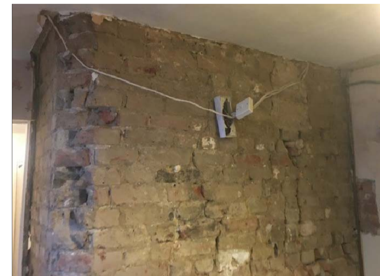
5 PHOTO OF EXISTING Elevation from sink room (upper portion)
