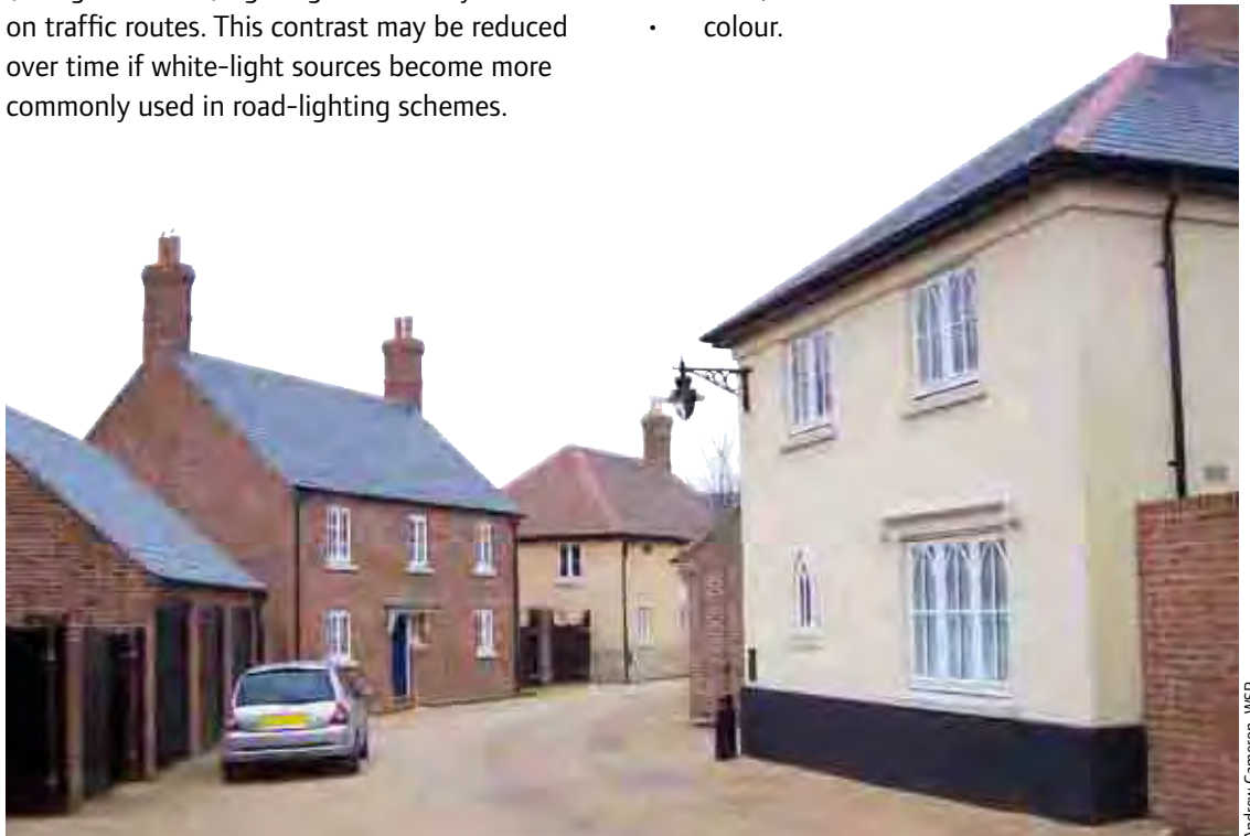
Figure 10.3 Street light mounted on a building.
