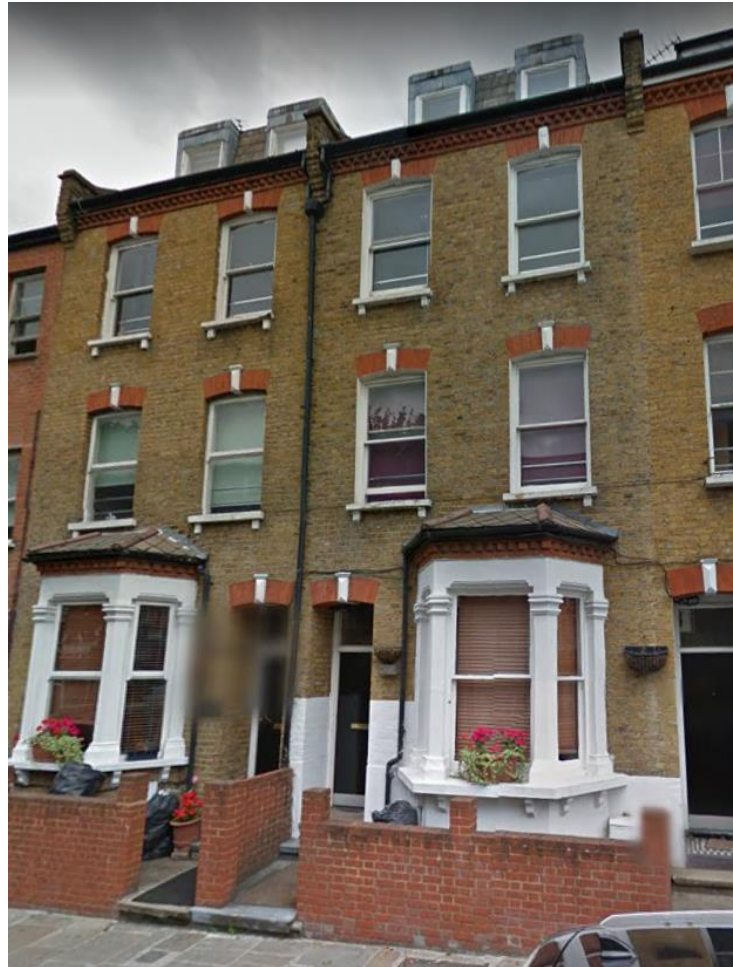
Figure 12: front of No 14 Fortess Road
