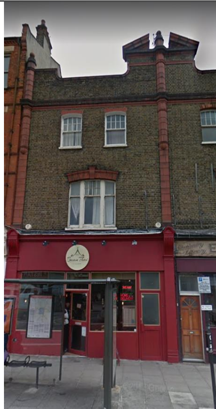
Figure 9: front of No 18 Fortess Road
