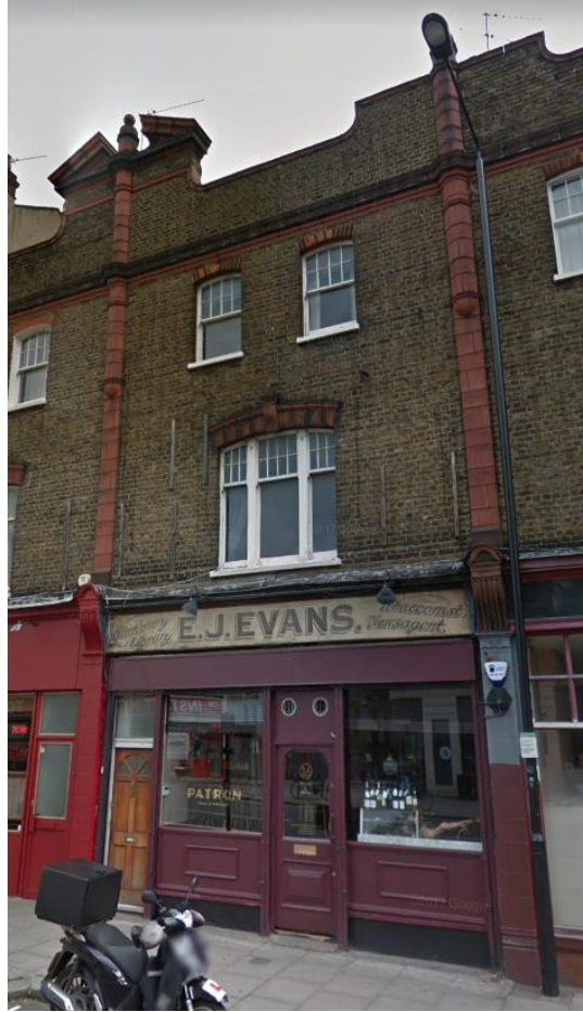
Figure 10: front of No 16 Fortess Road
