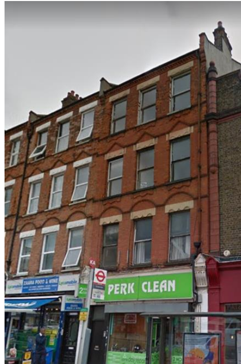
Figure 8: front of No 20 Fortess Road
