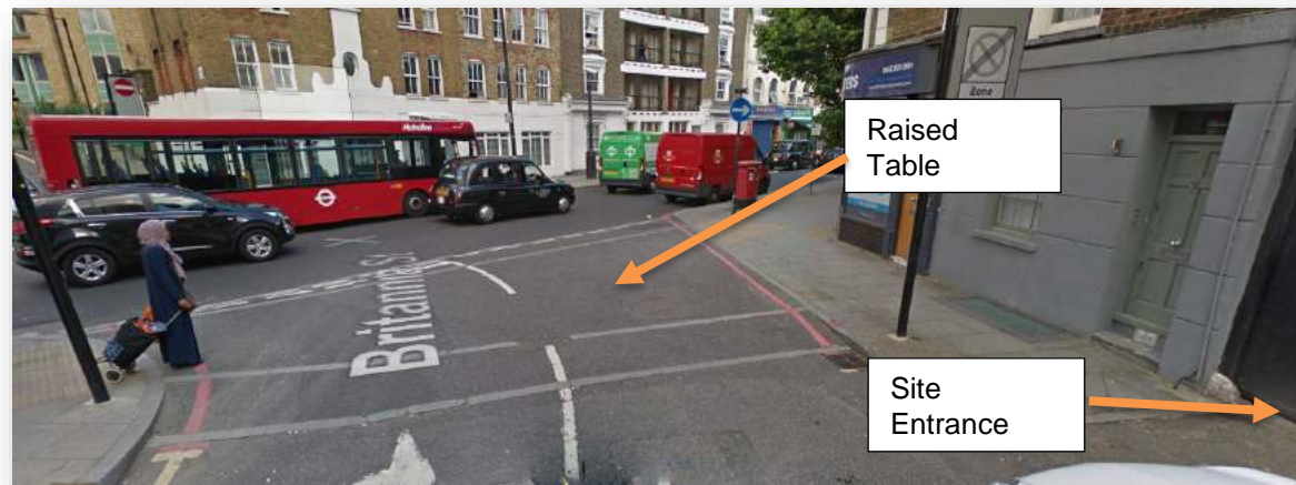
Figure 7.0 Raised Table forming barrier to surface water flow from Kings Cross Road
