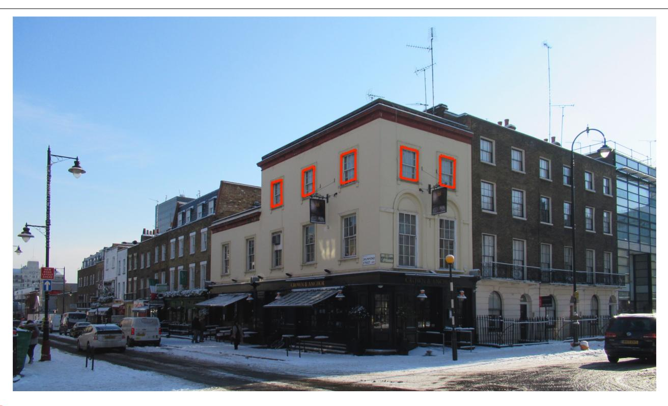
= Existing window openings where internal secondary glazing will be installed. The scope of secondary glazing work is limited to these openings only
