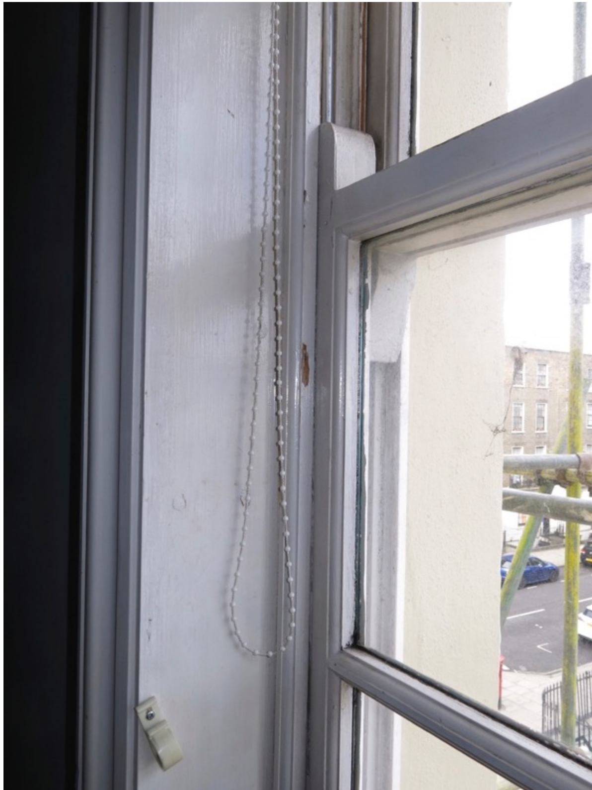
Figure 11. Detail of the window reveal to the bedroom windows. The existing window design and secondary glazing proposal is the same as the lounge
