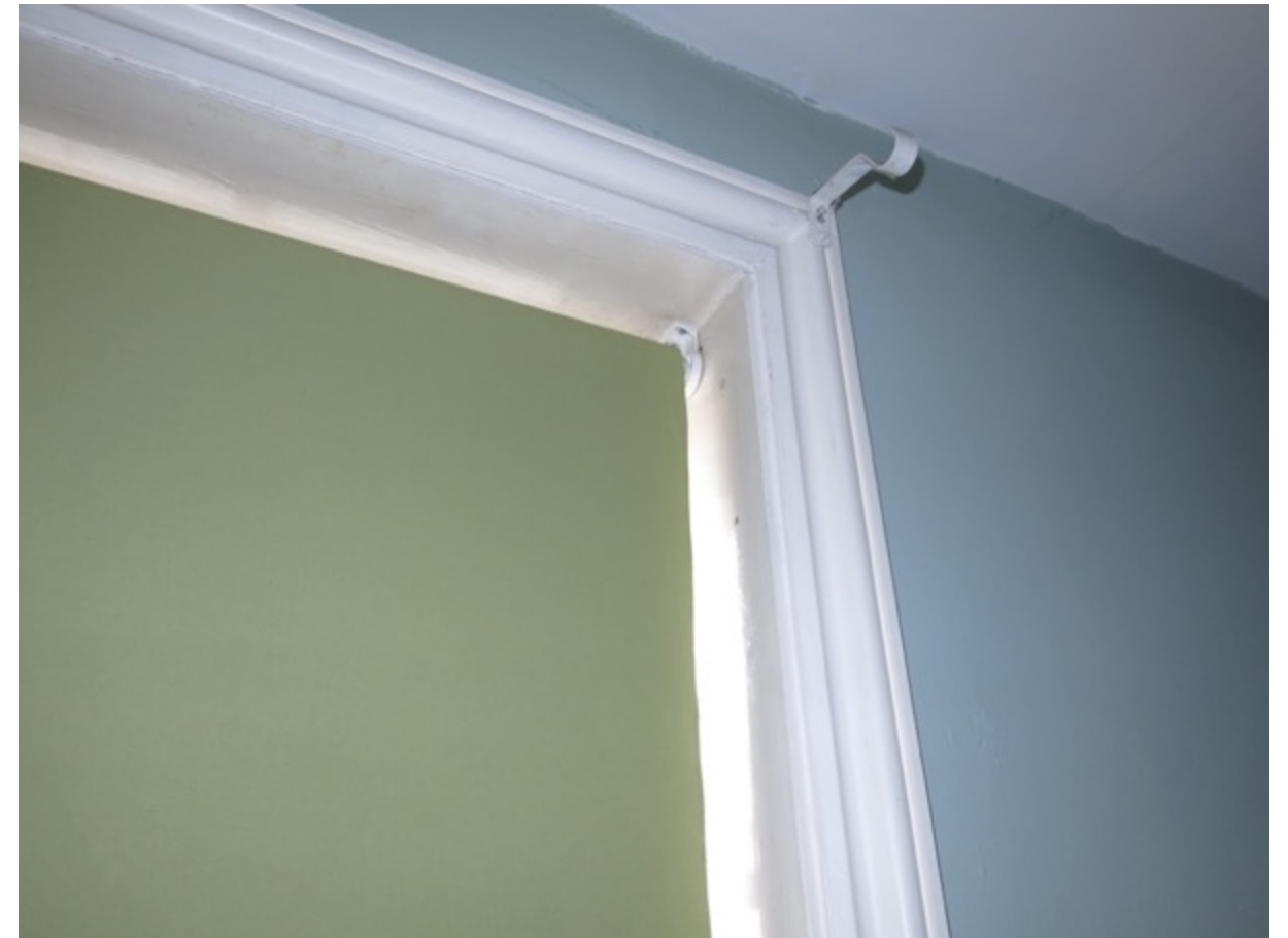
Figure 12. The window architrave and reveal
