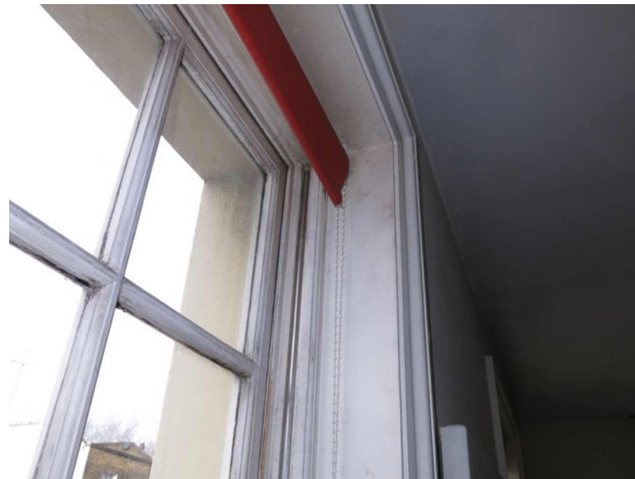
Figure 8. Detail of the existing upper sash, and window head in the lounge. The secondary glazing will sit within the existing window reveal depth
