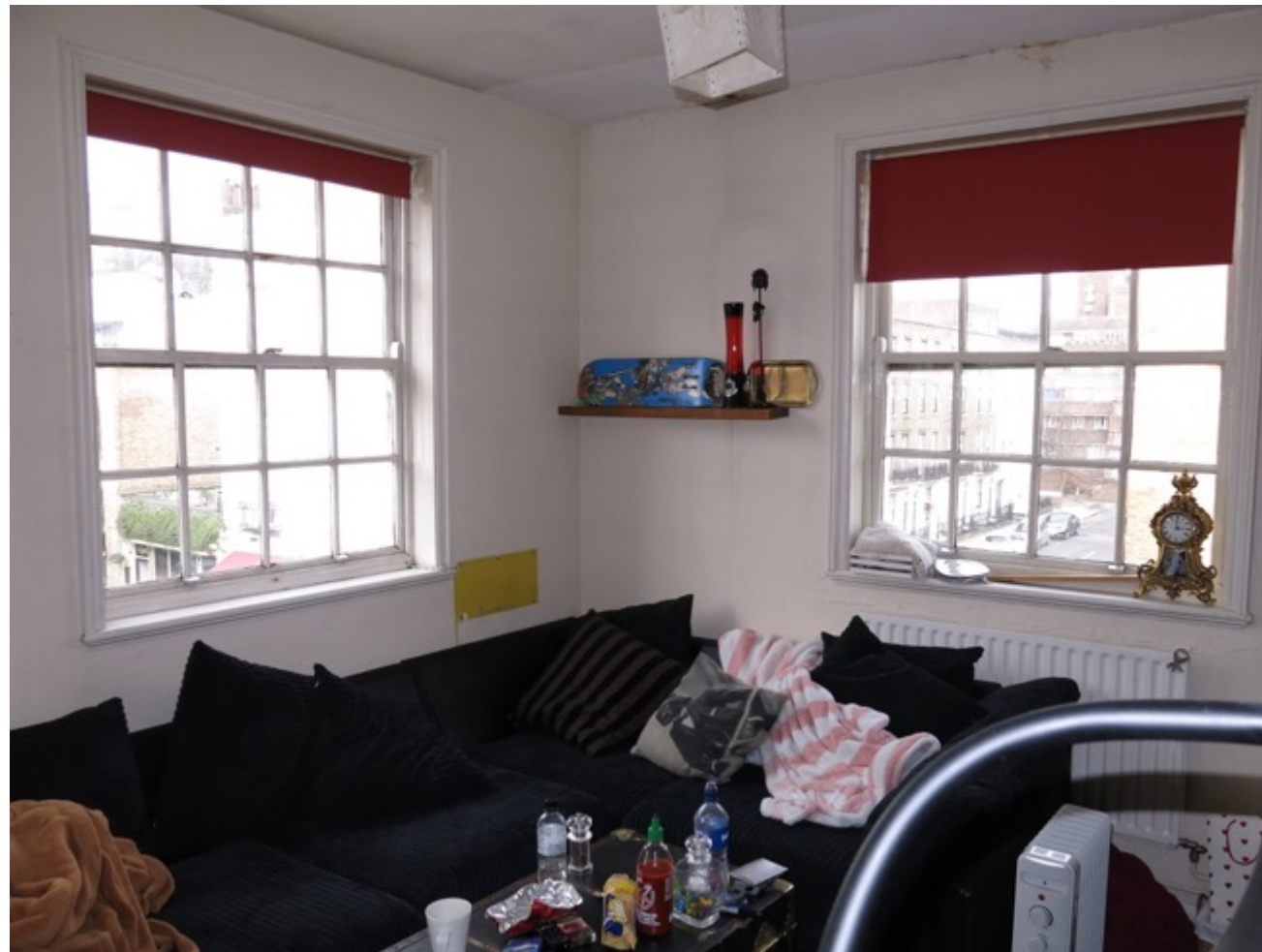
Figure 3. Internal view of two out of three of the lounge windows. The left hand one faces North Gower Street, the right one onto Drummond Street. The room has been completely replastered; the windows are modern replaces presumably replicating the originals
