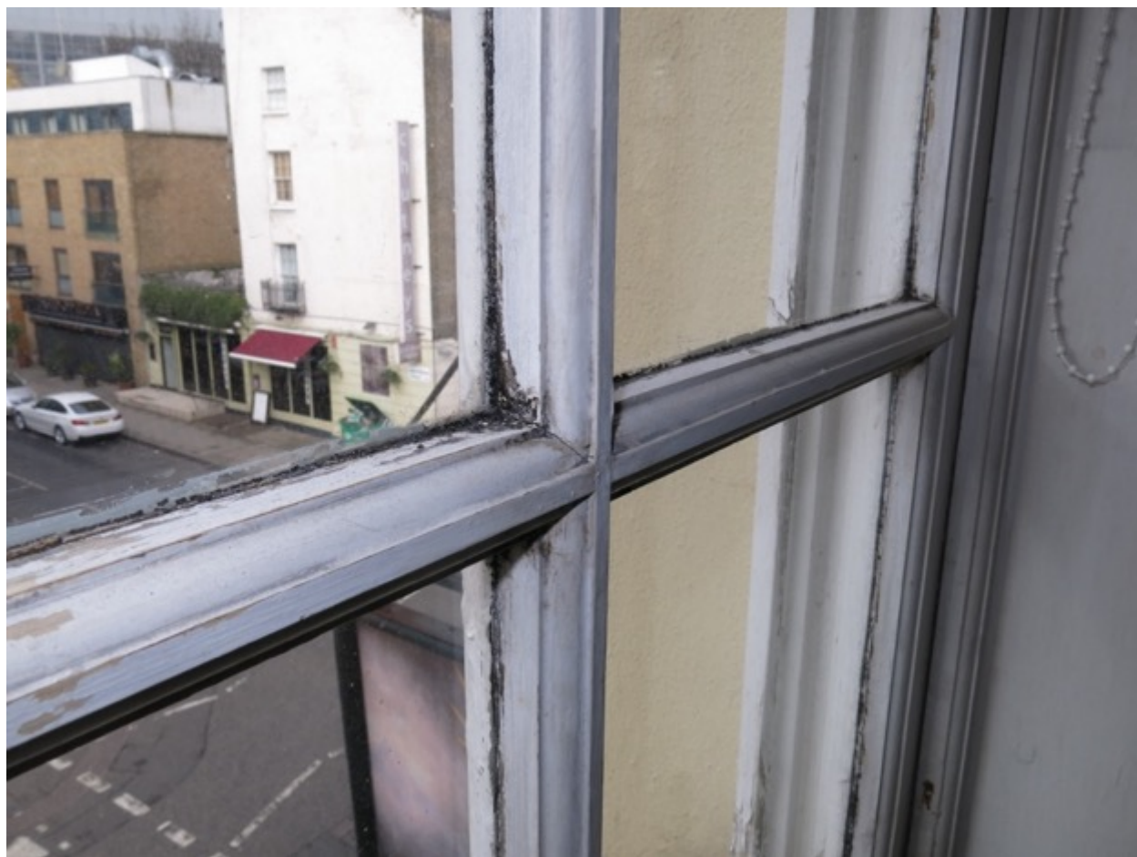
Figure 7. Detail of the existing lower sash, the glazing bars and single glazed 'float glass' in the lounge illustrating the sharp profiles and minimal paint. The windows are high quality modern replacements, presumably replicating the original window design
