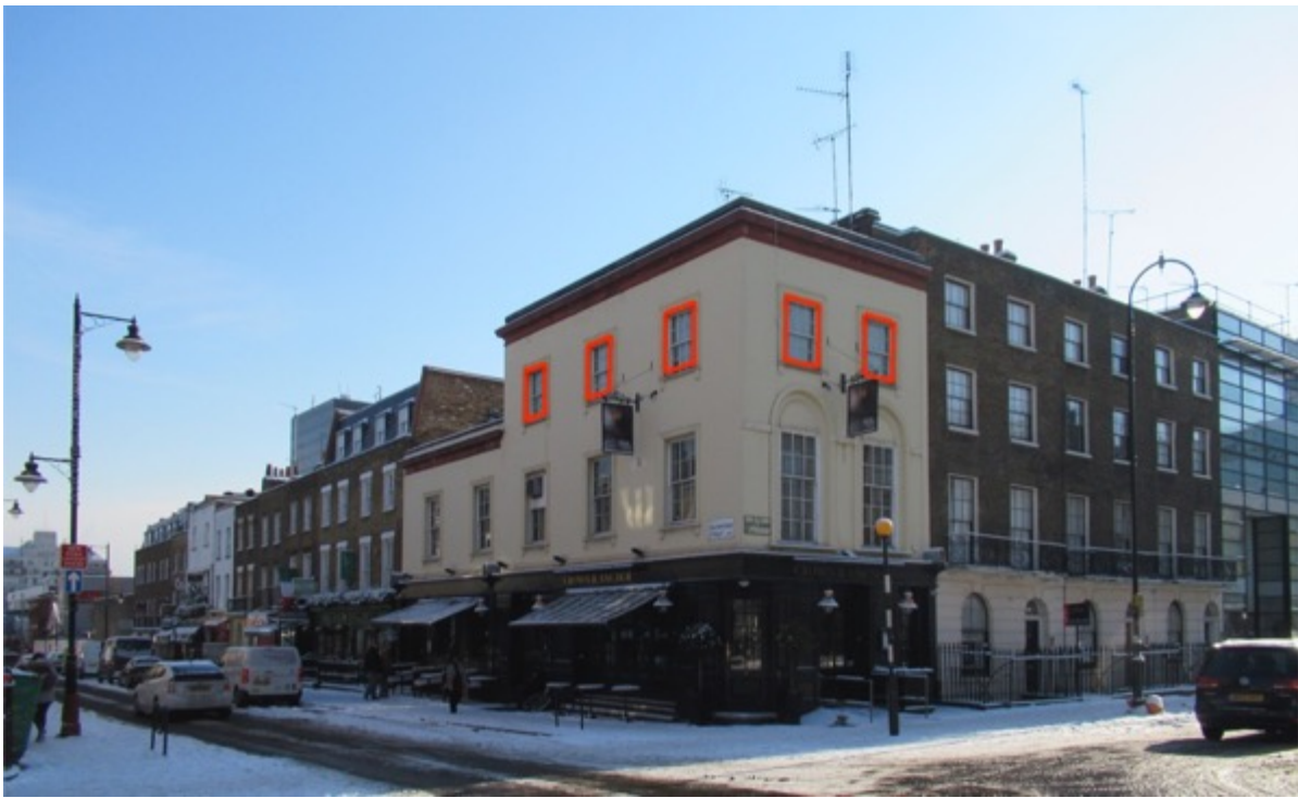
Figure 2: A view of the street facing elevations of the Crown and Anchor public house. Windows where internal secondary glazing will be installed are annotated in RED .
