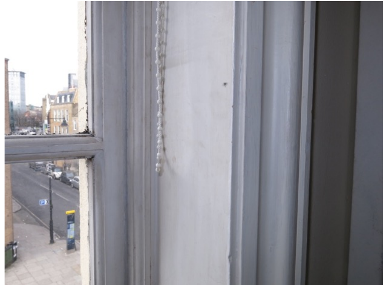
Figure 6. Detail of the existing timber window lining. The secondary glazing will fit into the window reveal and screw fix to these window linings
