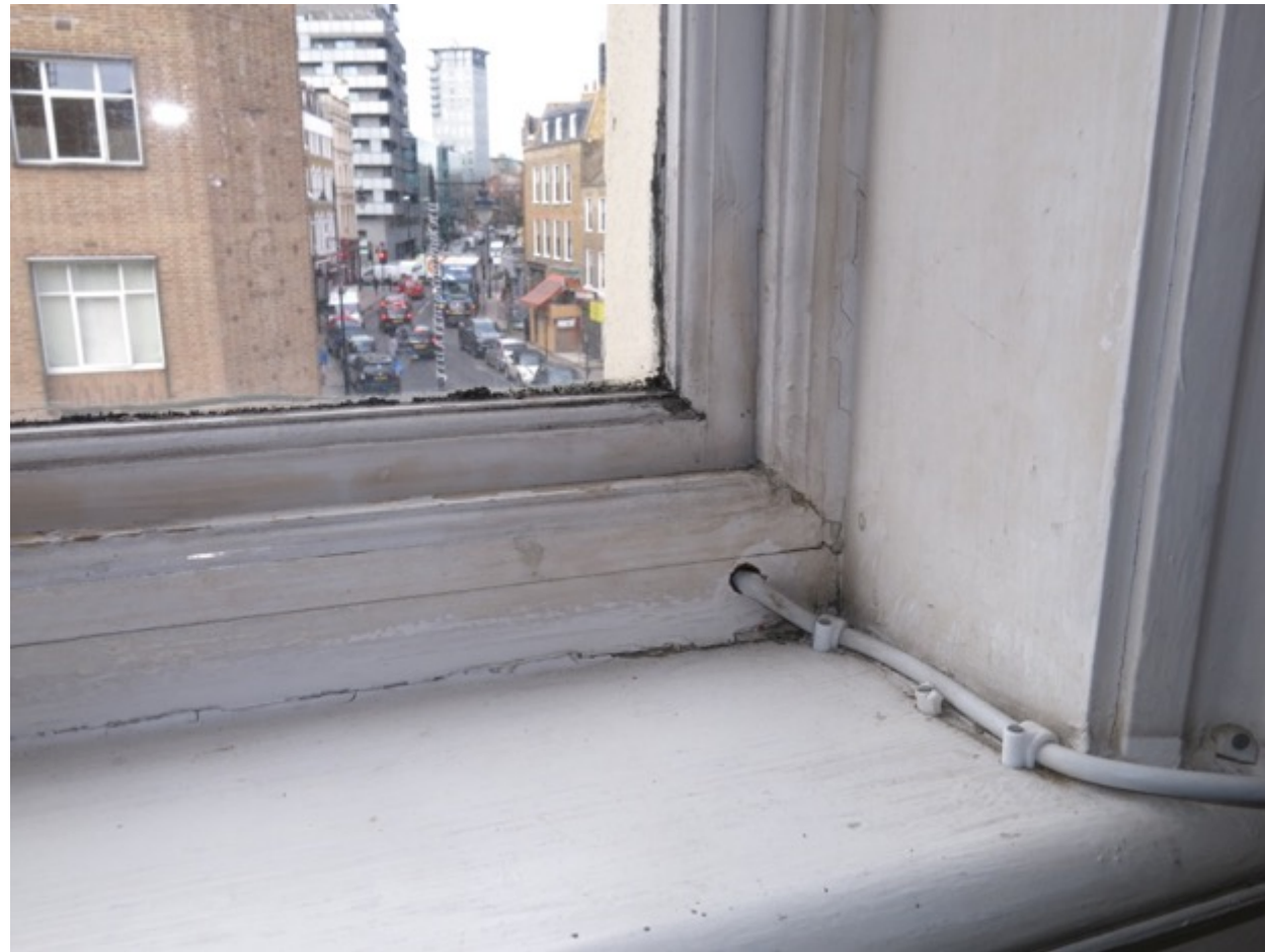
Figure 5. Detail of the existing window cill board in the lounge. The secondary glazing will sit onto this existing cill board
