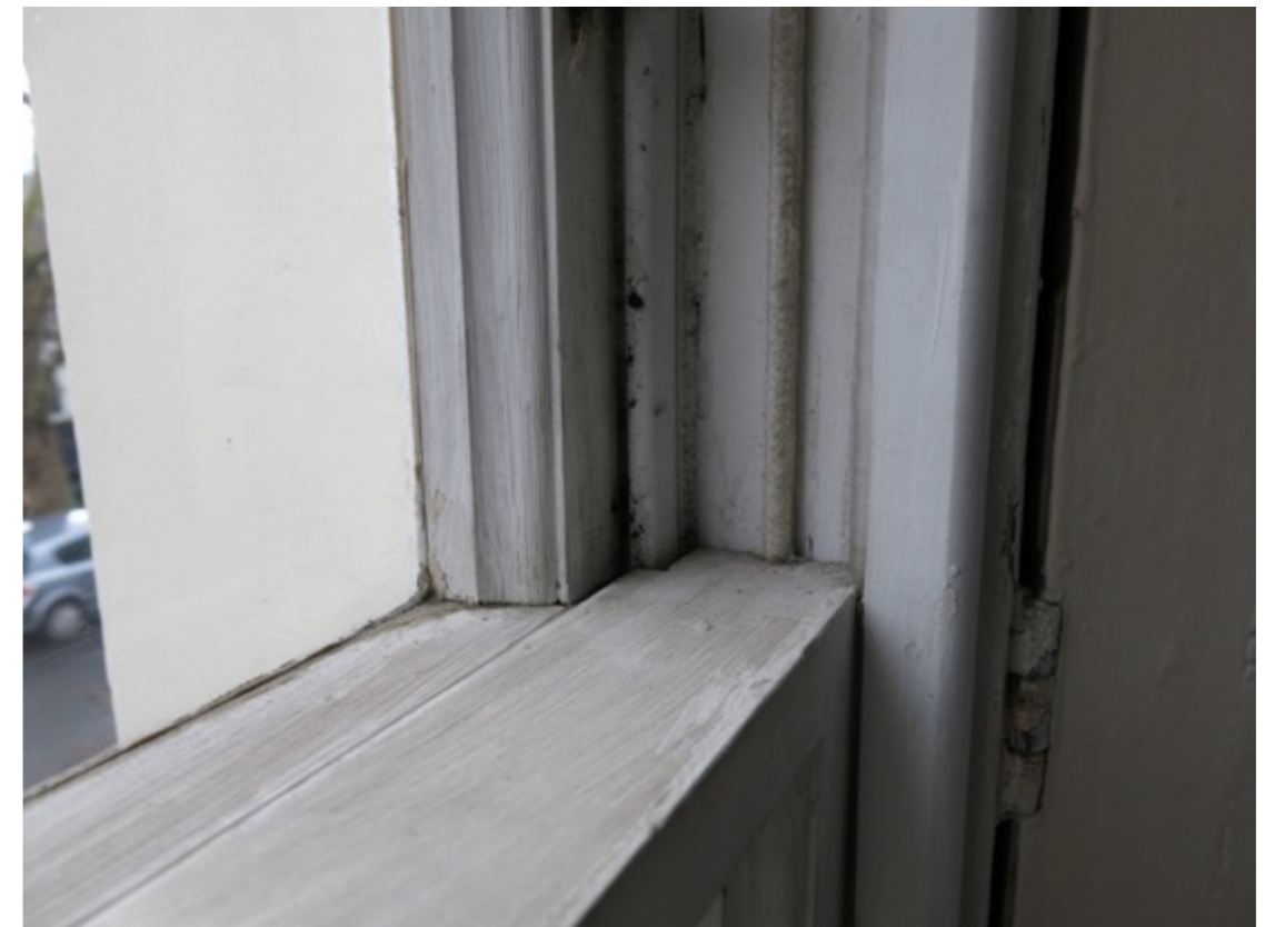
Figures 15 and 16: Detail of the replacement window sash and glazing bars illustrating the traditional 'lamb's tongue' moulding and minimal paint covering. The first floor balcony is located immediately outside
