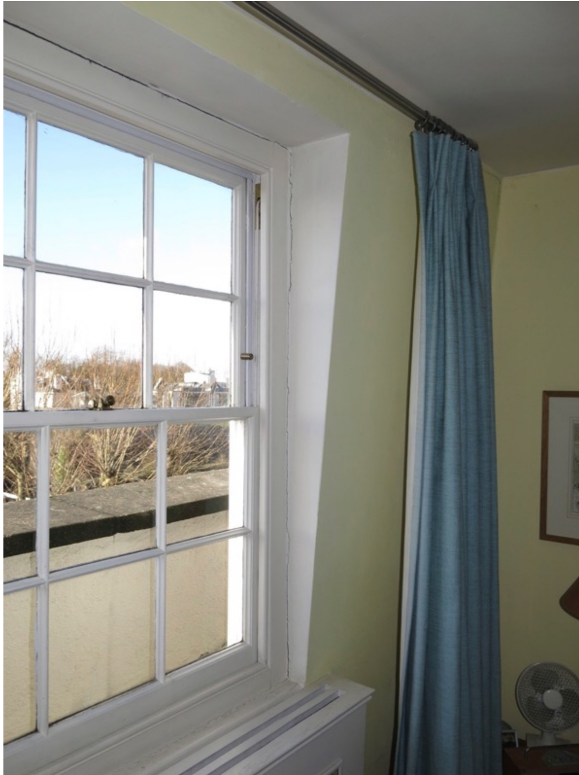
Figure 26: View of the window with dormer cheek and reveal
