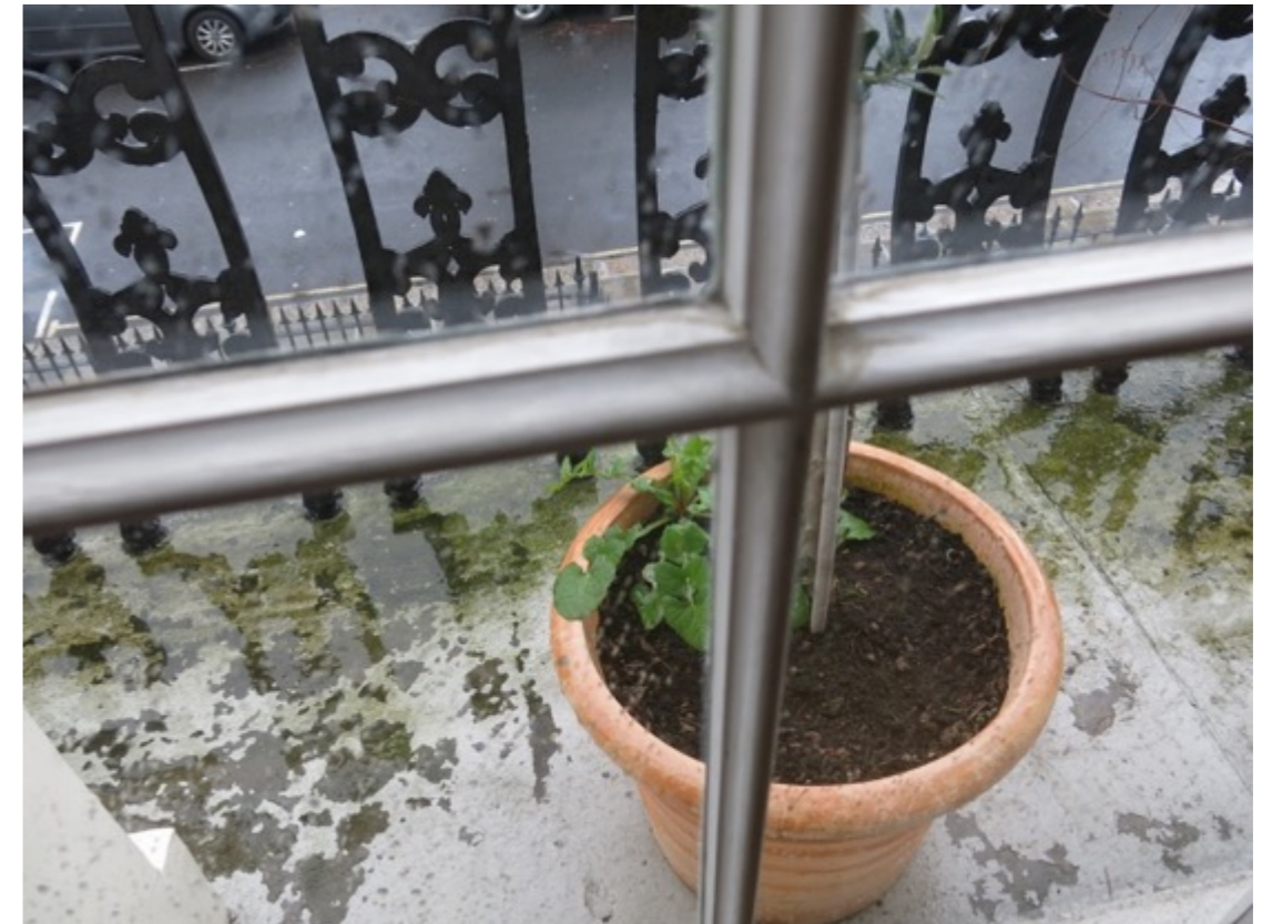
Figures 15 and 16: Detail of the replacement window sash and glazing bars illustrating the traditional 'lamb's tongue' moulding and minimal paint covering. The first floor balcony is located immediately outside
