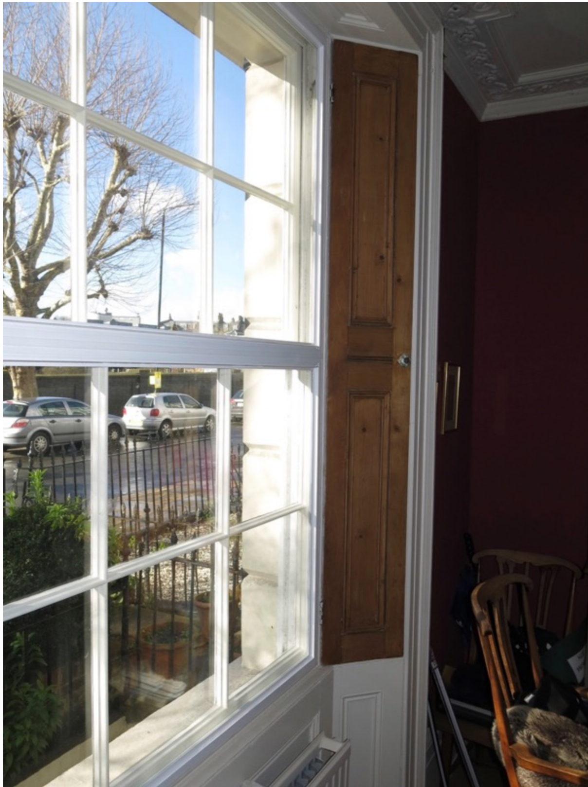
Figure 10: Sash window with secondary glazing installed on the staff bead allowing the shutters to close
