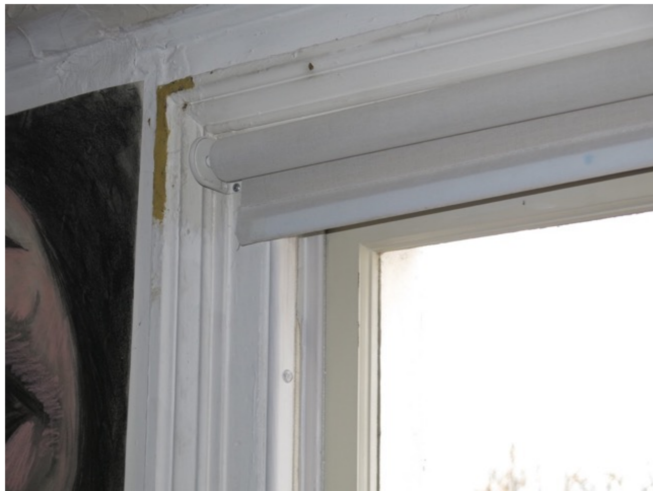
Figure 22: Existing window head and architrave
