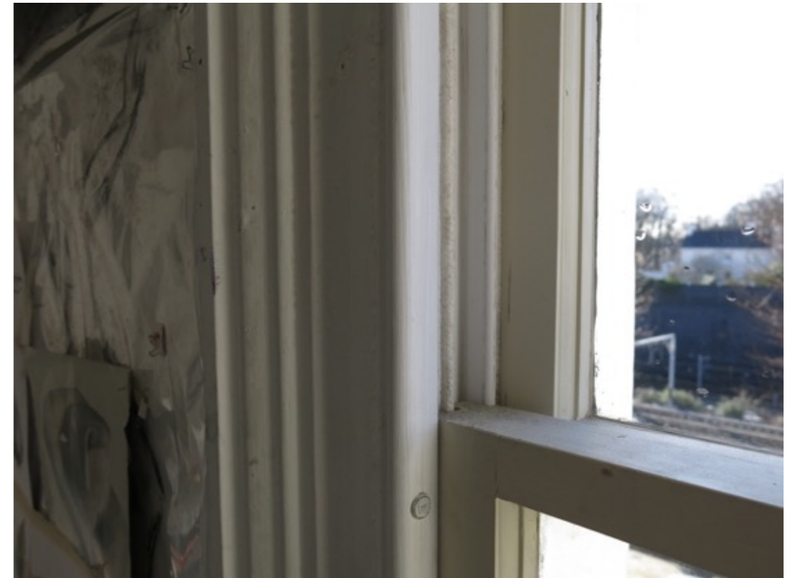
Figures 20 and 21: New window sashes and staff bead to original/period design
