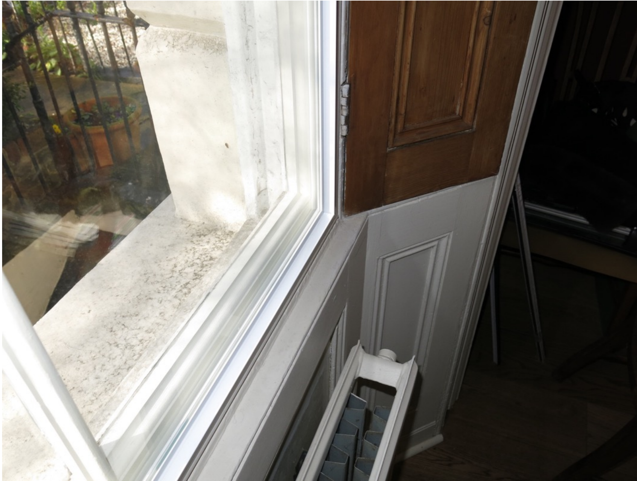
Figure 12: View looking at the window sill illustrating the close proximity of the radiator below. Note the alignment of the secondary glazing allowing the shutters to close.
