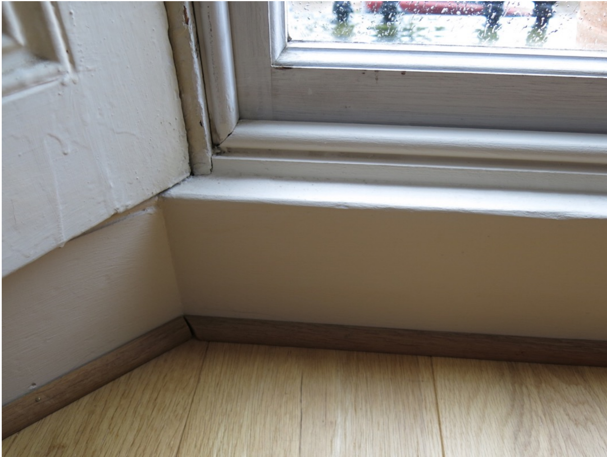
Figure 17: The window cill and floor with window shutter in the left of the photograph. Secondary glazing will sit onto the floor to support the weight
