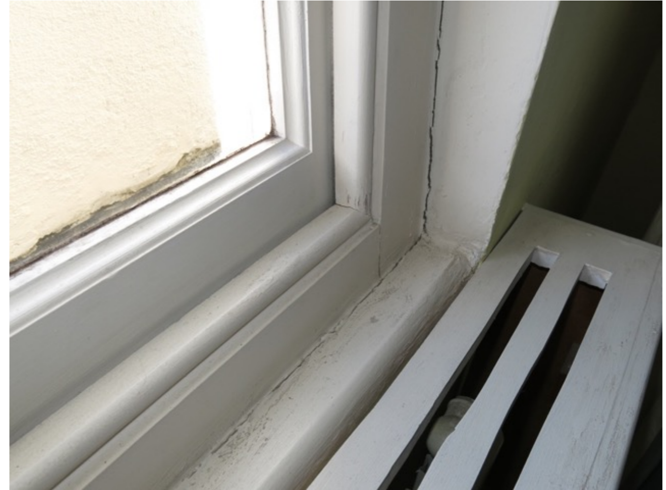
Figure 27: Window cill with radiator in front. The window sash and staff bead have been replaced
