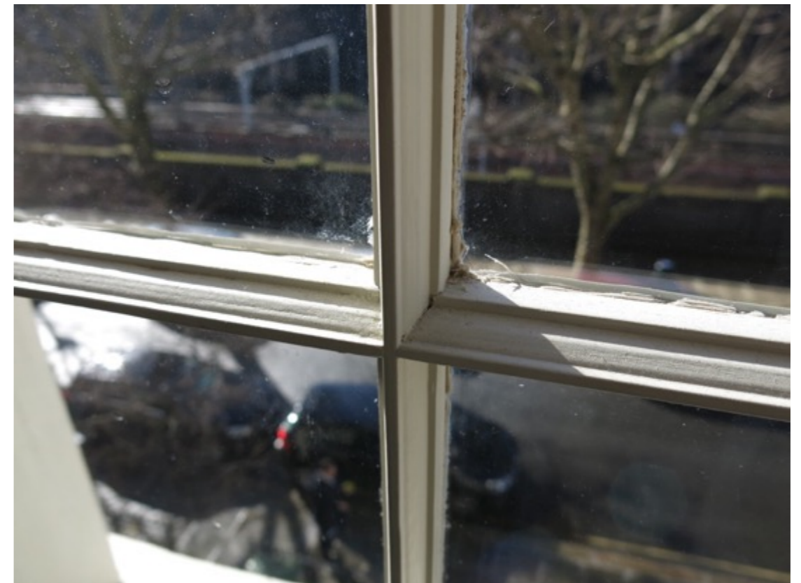
Figures 20 and 21: New window sashes and staff bead to original/period design
