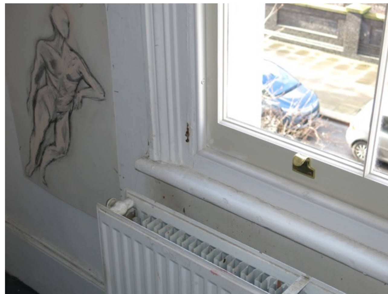
Figure 23: Existing window cill and architrave
