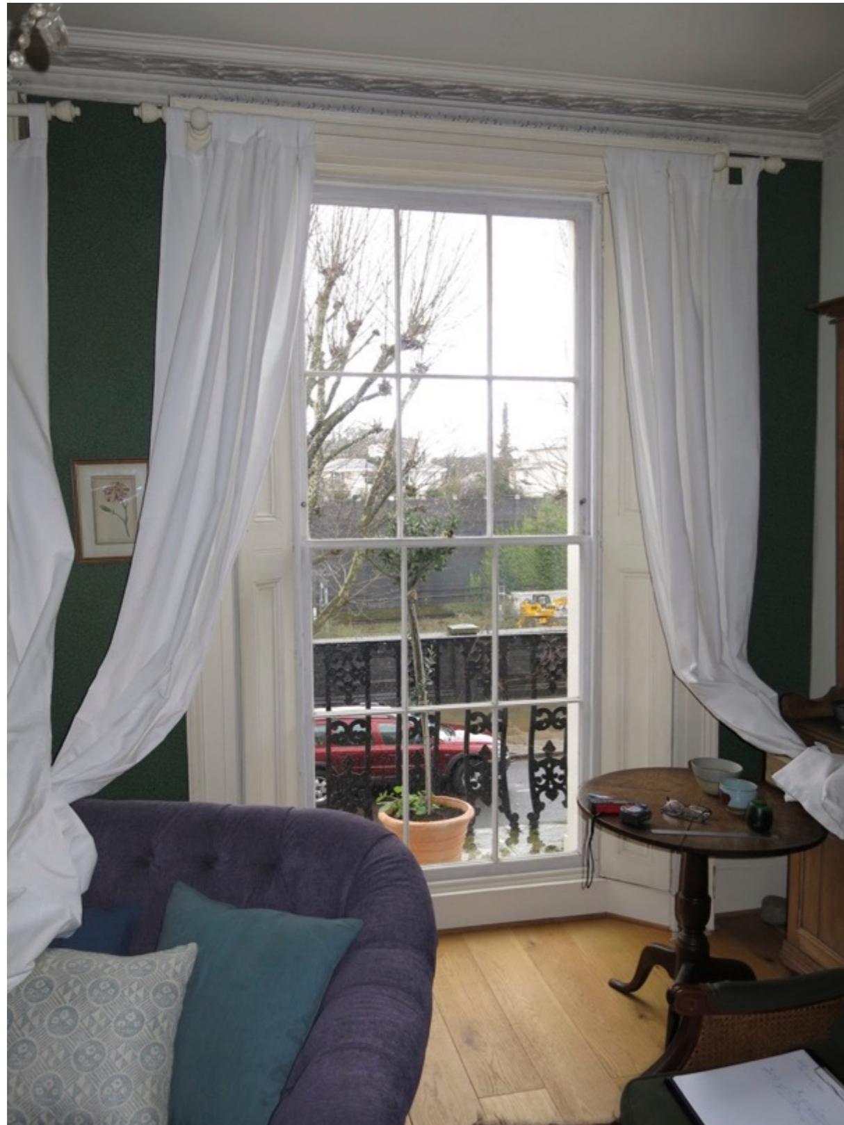
Figure 14: Almost full height sash window with shutters opening out onto the continuous Mornington Terrace balcony
