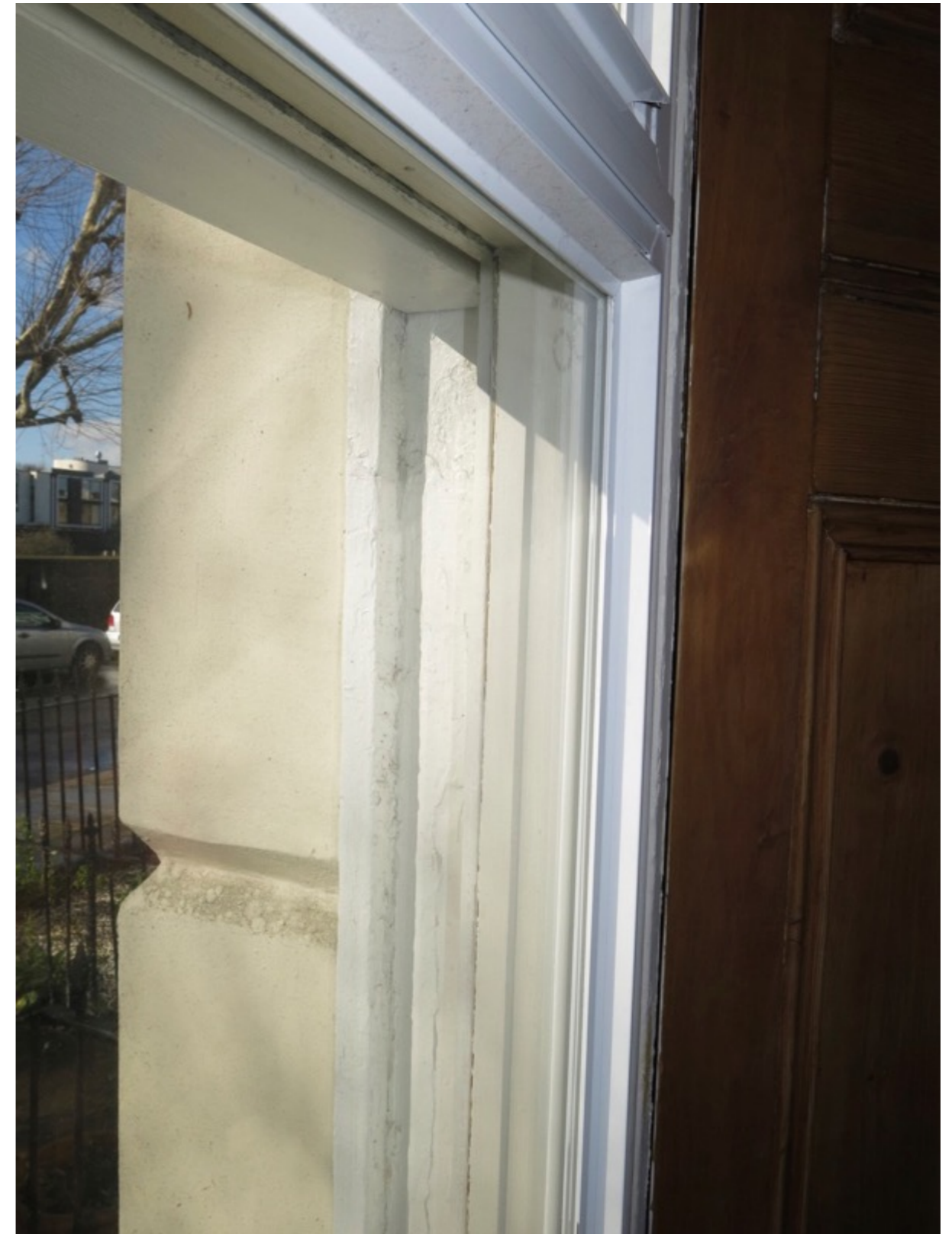
Figure 11: Detail of the secondary glazing illustrating the low profile and unobtrusive appearance
