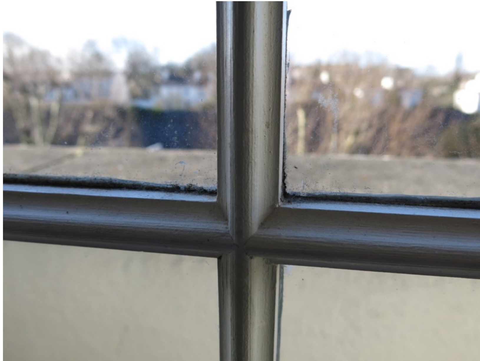
Figure 28: Detail of the glazing bars to one of the replacement sashes
