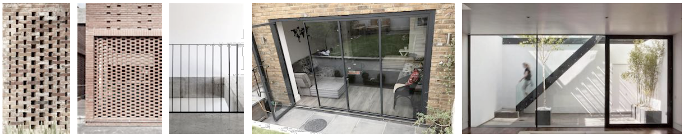
Perforated brick screen
