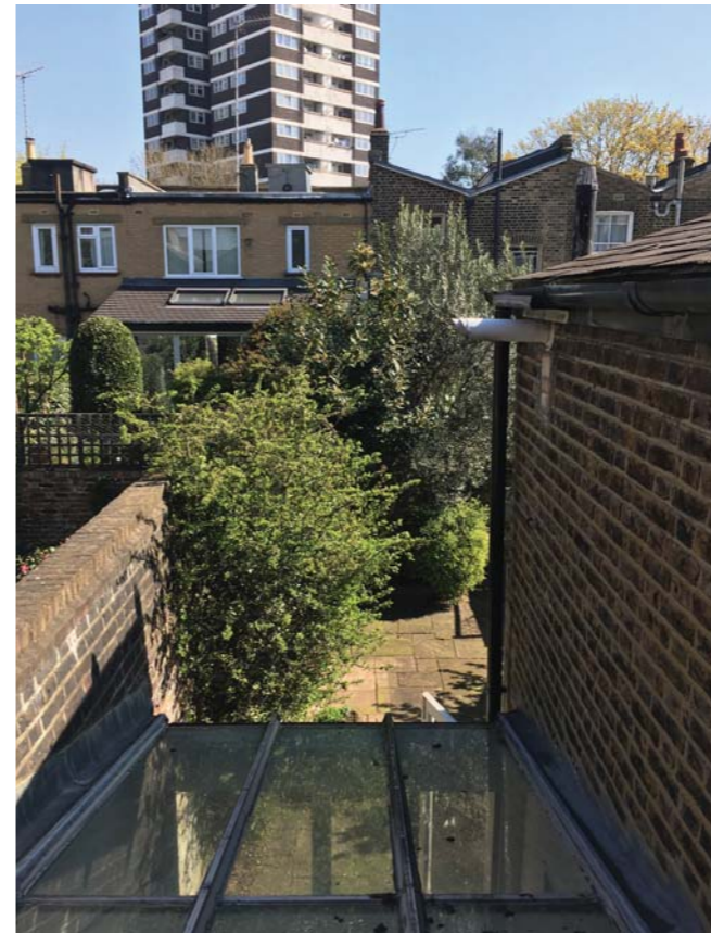
View from first floor over conservatory
