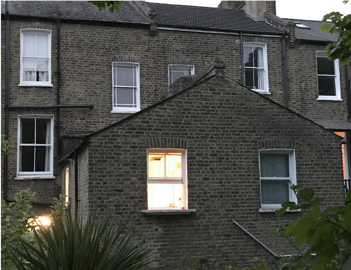
3. View of rear elevation
