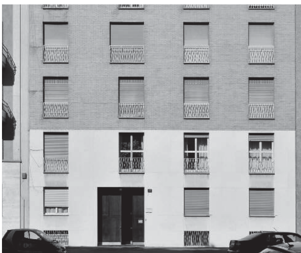
Residential Building, Milan: Asnago & Vender: Materially Defined Base & Top
