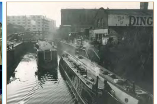
TRANSPORT & WAREHOUSING: Camden Town
