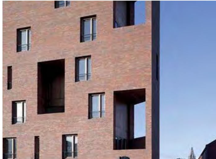
Timberyard Housing, O'Donnell & Tuomey: Double Height Openings
