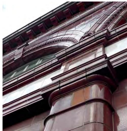
Chalk Farm Station: Detail of Curved Faience Blocks & Arches
