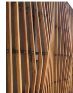
Timber play fence
