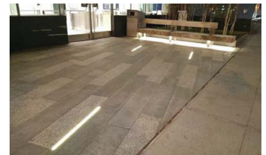
Pavers with integrated feature lighting
