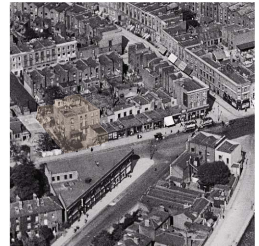
Aerial photograph of 18-22 Haverstock Hill (coloured brown) from 1920s
