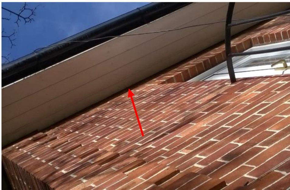
Figure 2: Gap between soffit and brickwork
