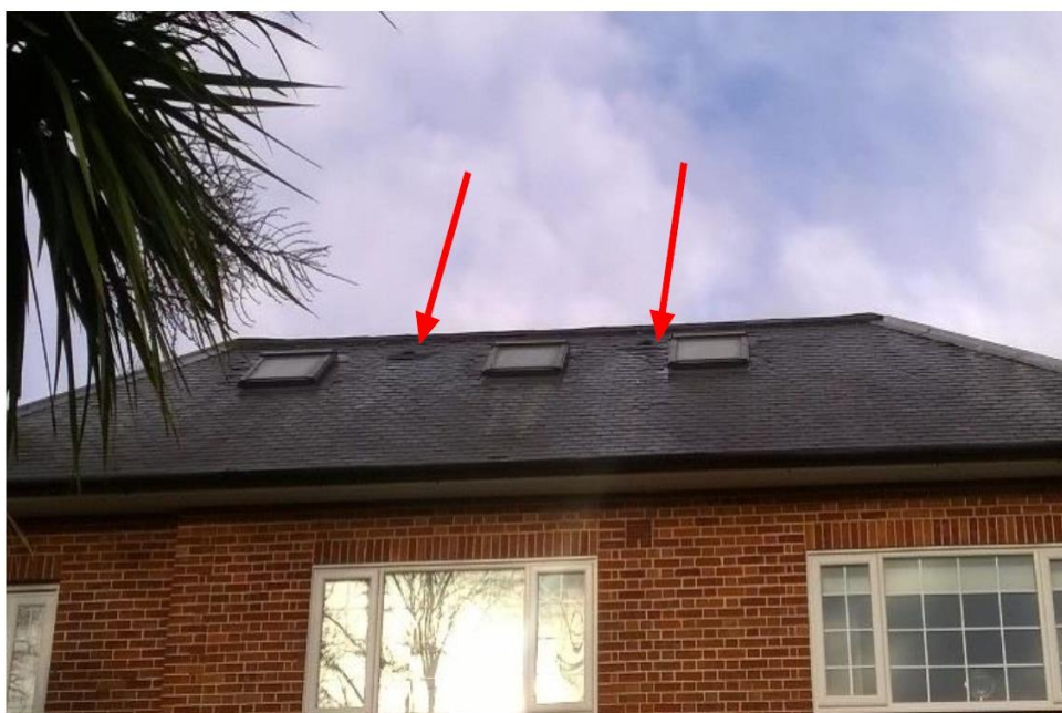
Figure 1: Missing and slipped tiles on southern elevation
