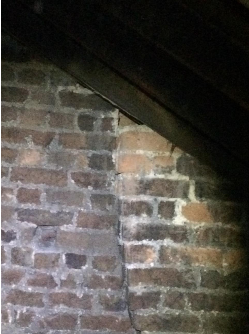
Photograph 13 – Internal roof void
