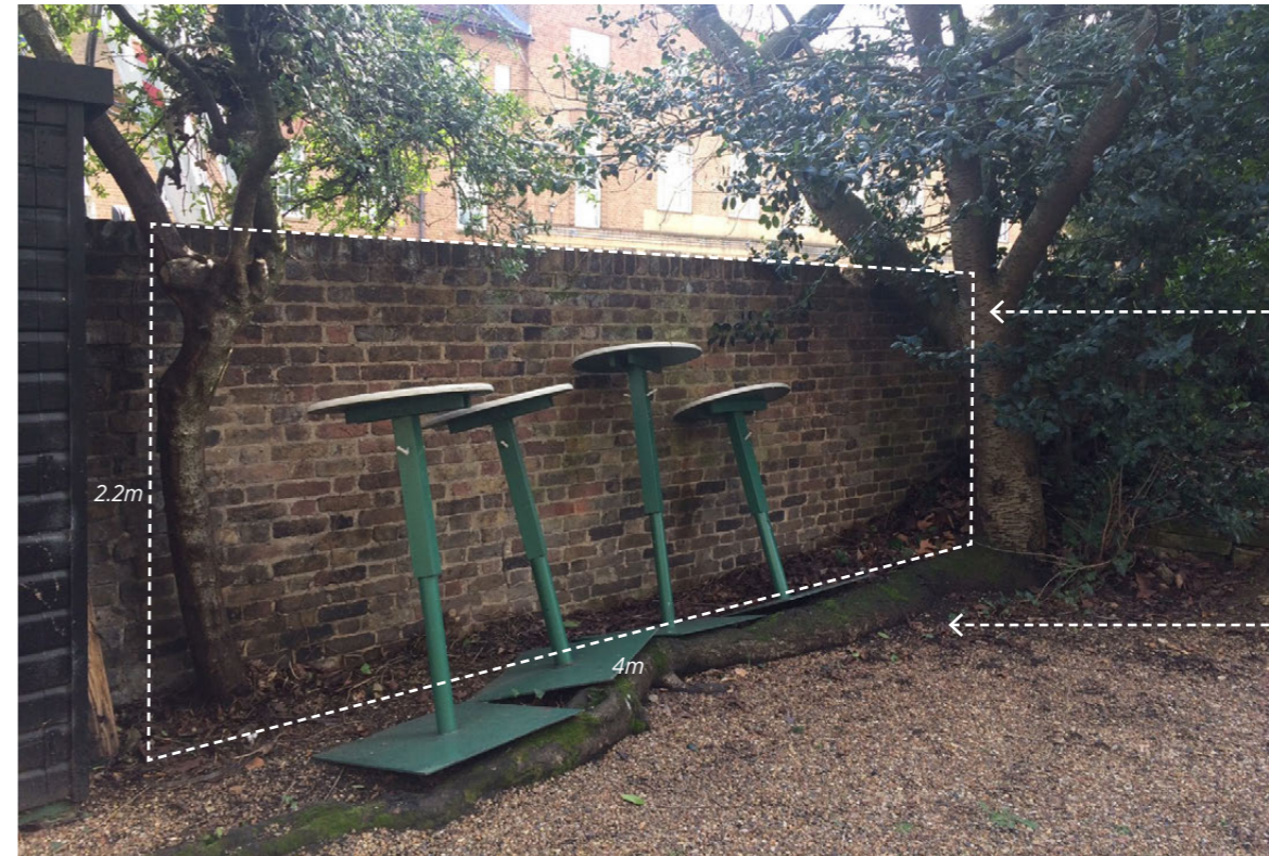
Church yard elevation
