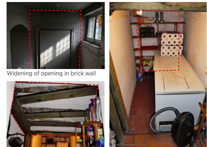
Remove stair treads above.
