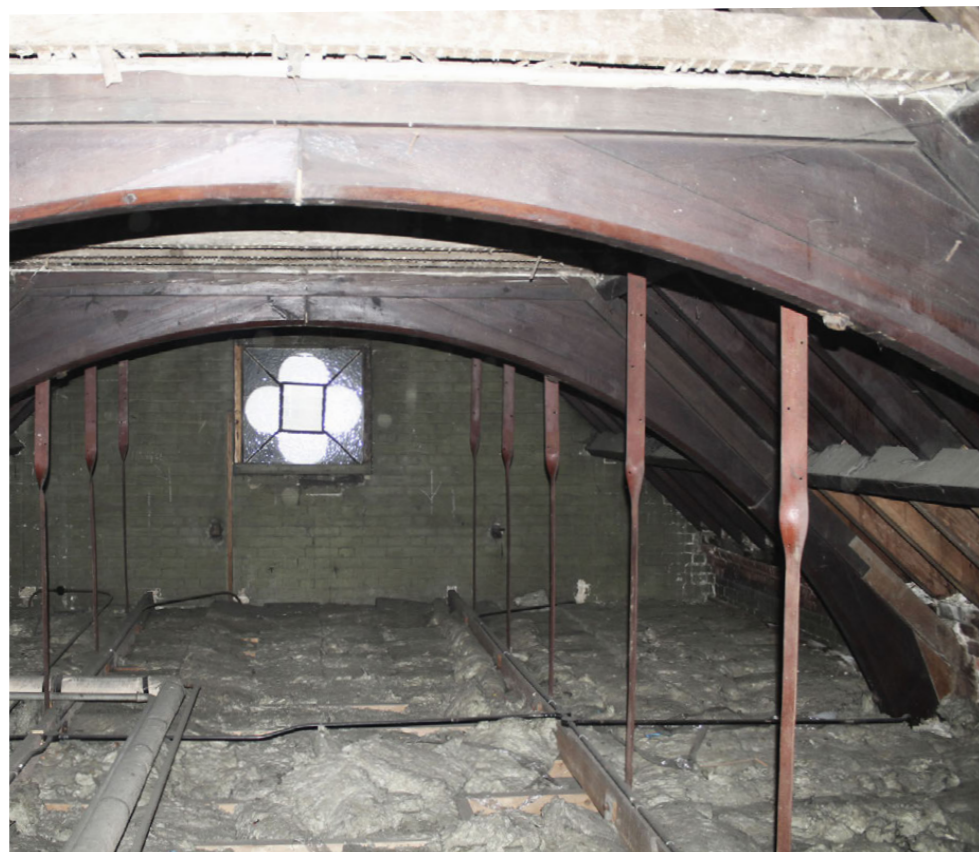
④ Existing wooden roof trusses and rose window in roof attic
