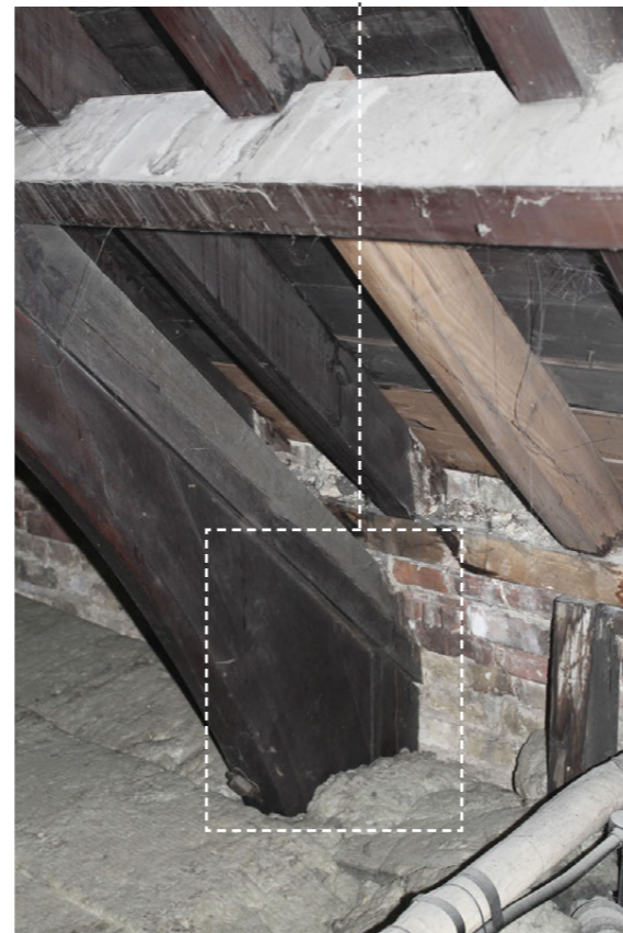
Truss connection to brick wall
