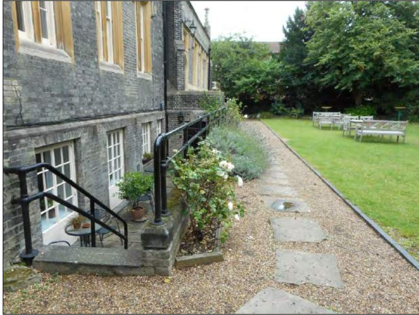
Plate 7: View of area for proposed sunken terrace to extend from existing basement level
