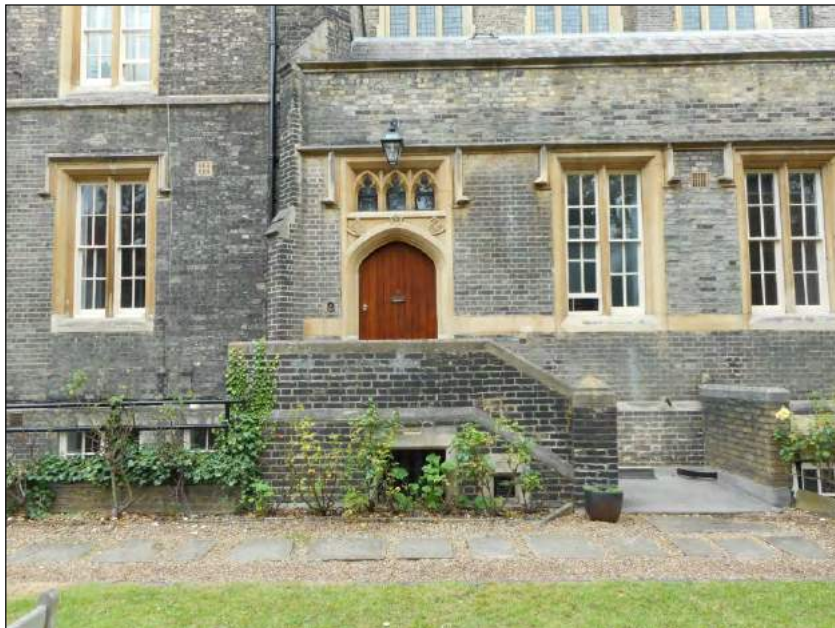
Plate 8: View of existing staircase leading to Nos 4 and 5 St Katharine's Precinct
