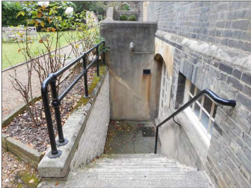
Plate 6: View of access to basement level on the eastern side of Nos 4 and 5 St Katharine's Precinct
