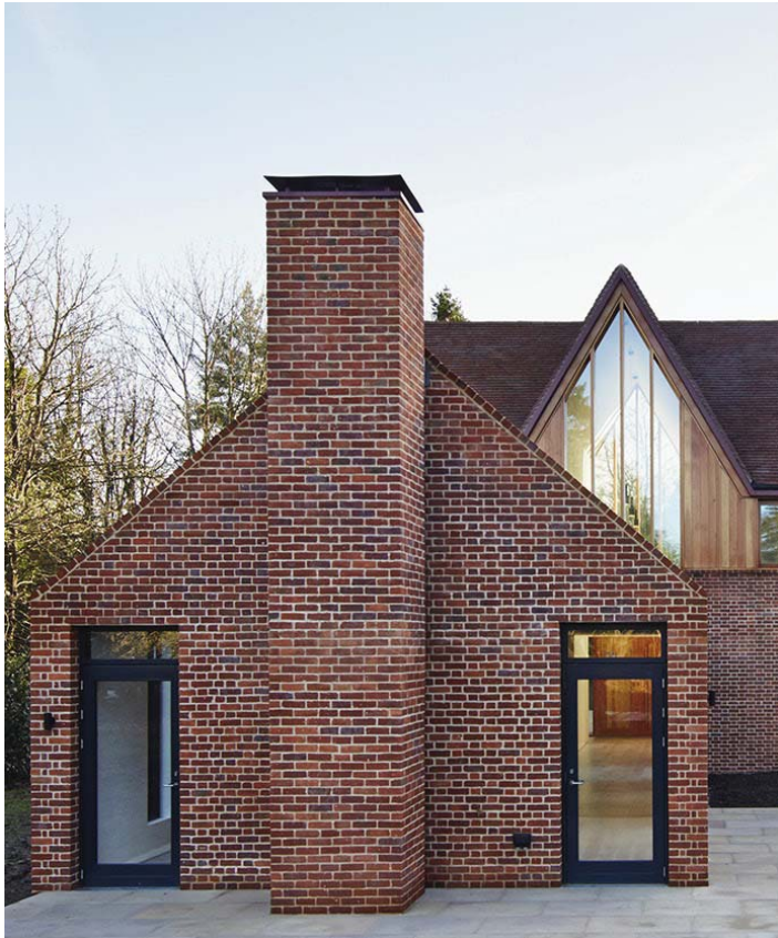
Pennycroft by Napier Clark architects
