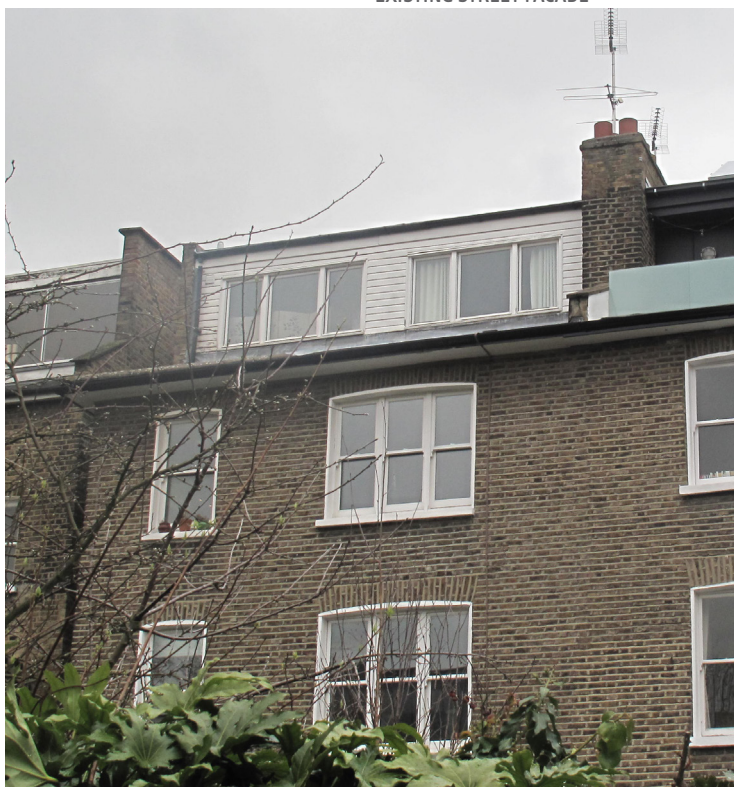
EXISTING REAR FACADE
