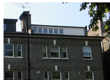
EXISTING STREET FACADE
