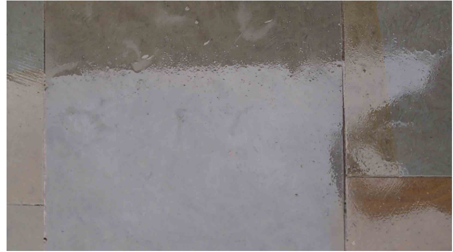
High-quality York stone pavement, Ely Place
