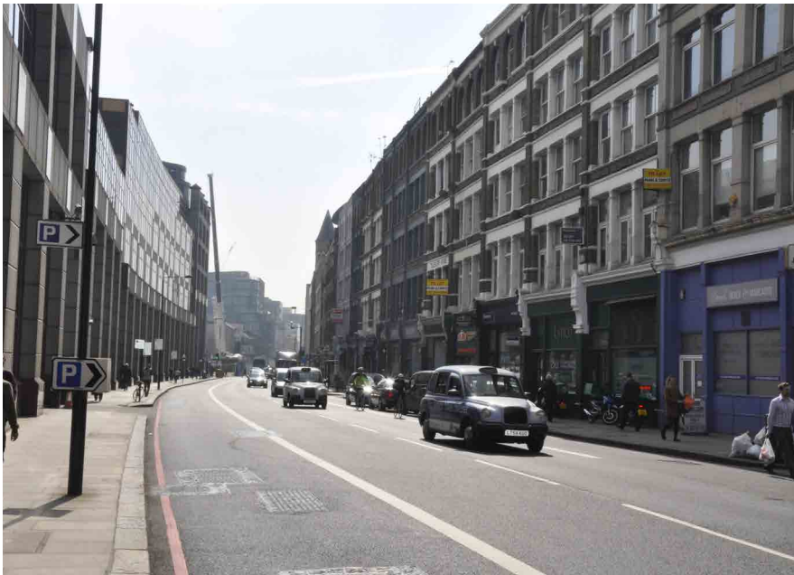
Farringdon Road, looking south, showing Nos 39-73 (Positive) on the right
