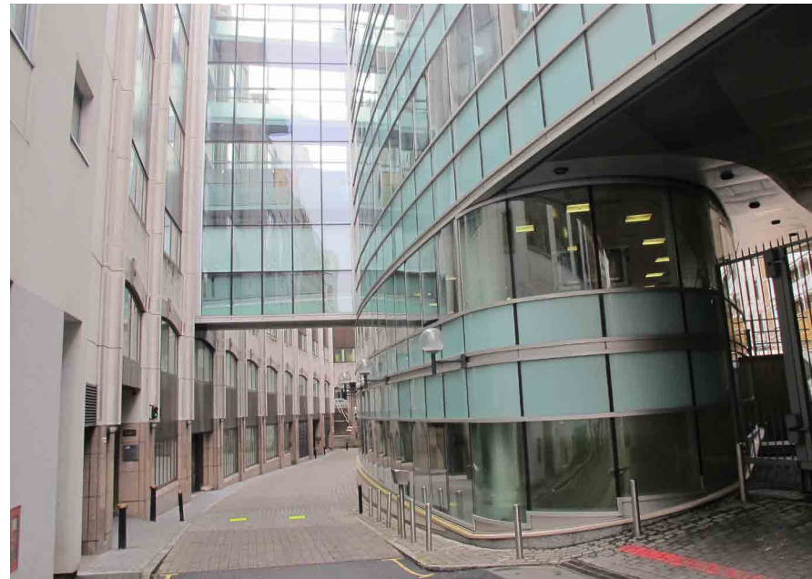
South end of Saffron Hill, showing rear of 17 Charterhouse Street
