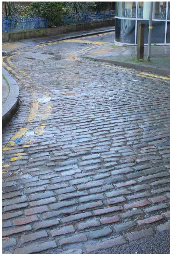
Intact roadway of granite setts, Poole's Buildings, Mount Pleasant
