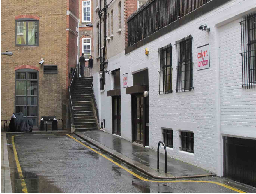
Painted brickwork, Vine Hill
