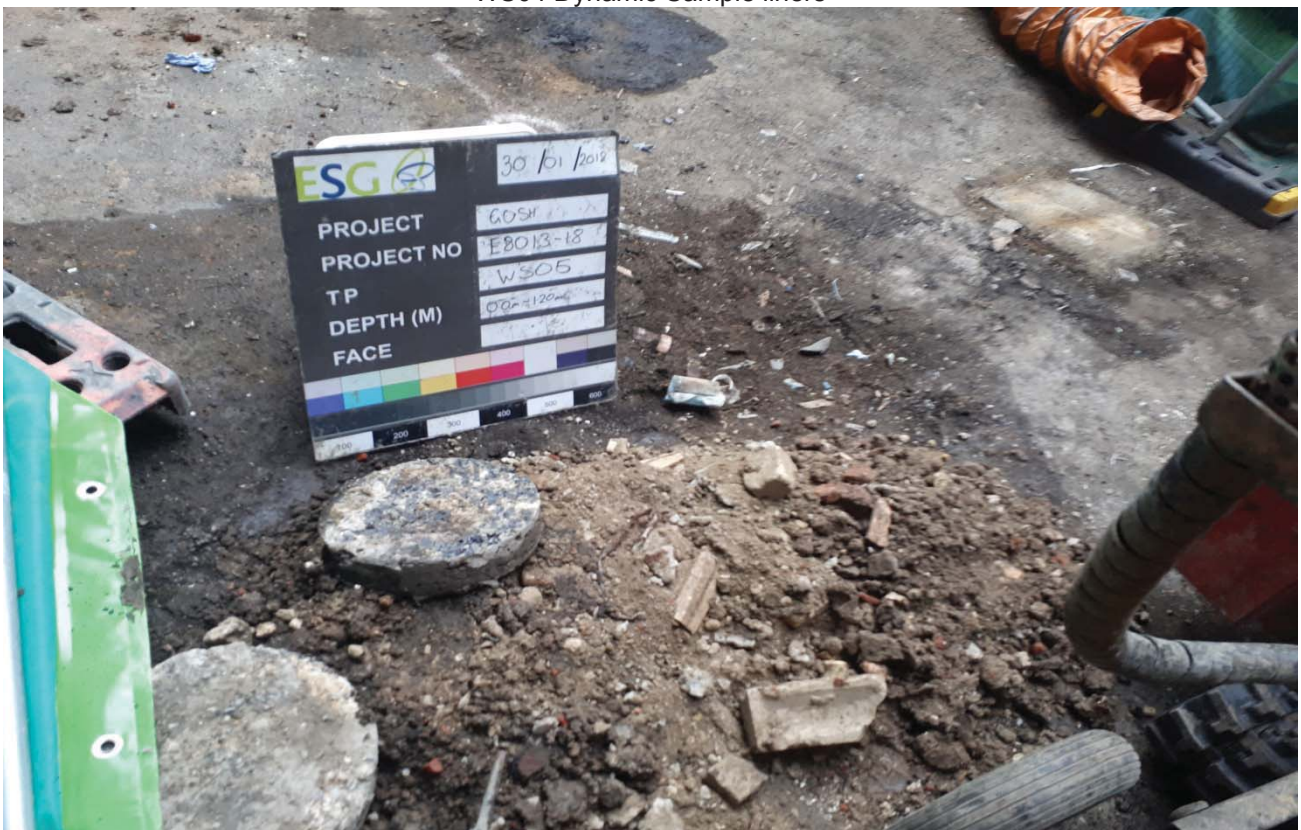
WS05 Concrete Core
