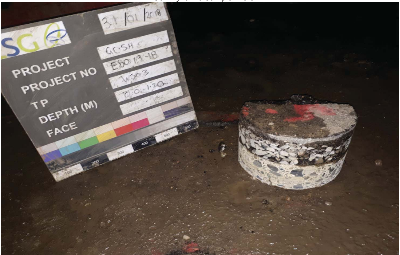
WS03 Concrete Core
