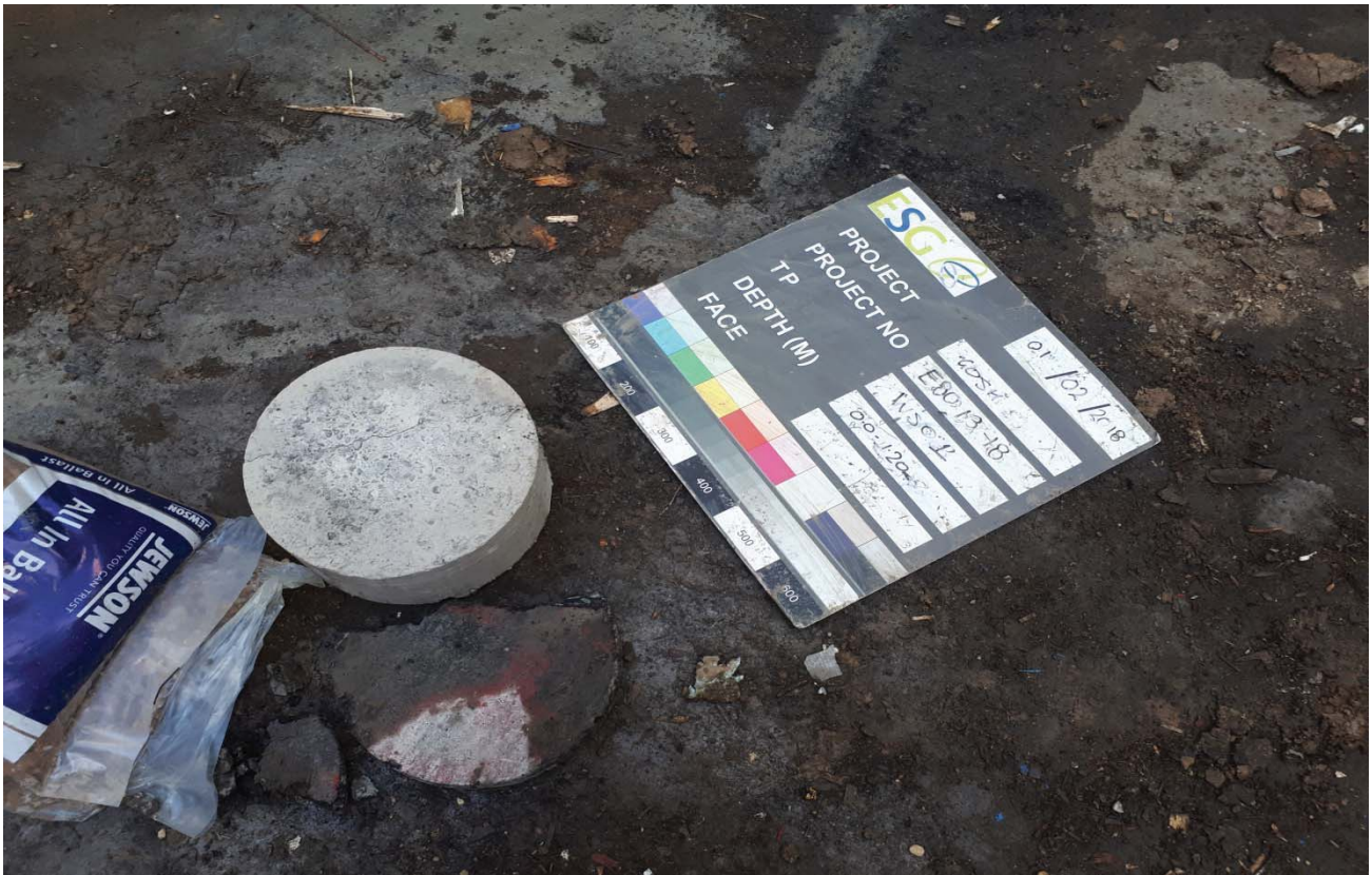
WS01 Concrete core
