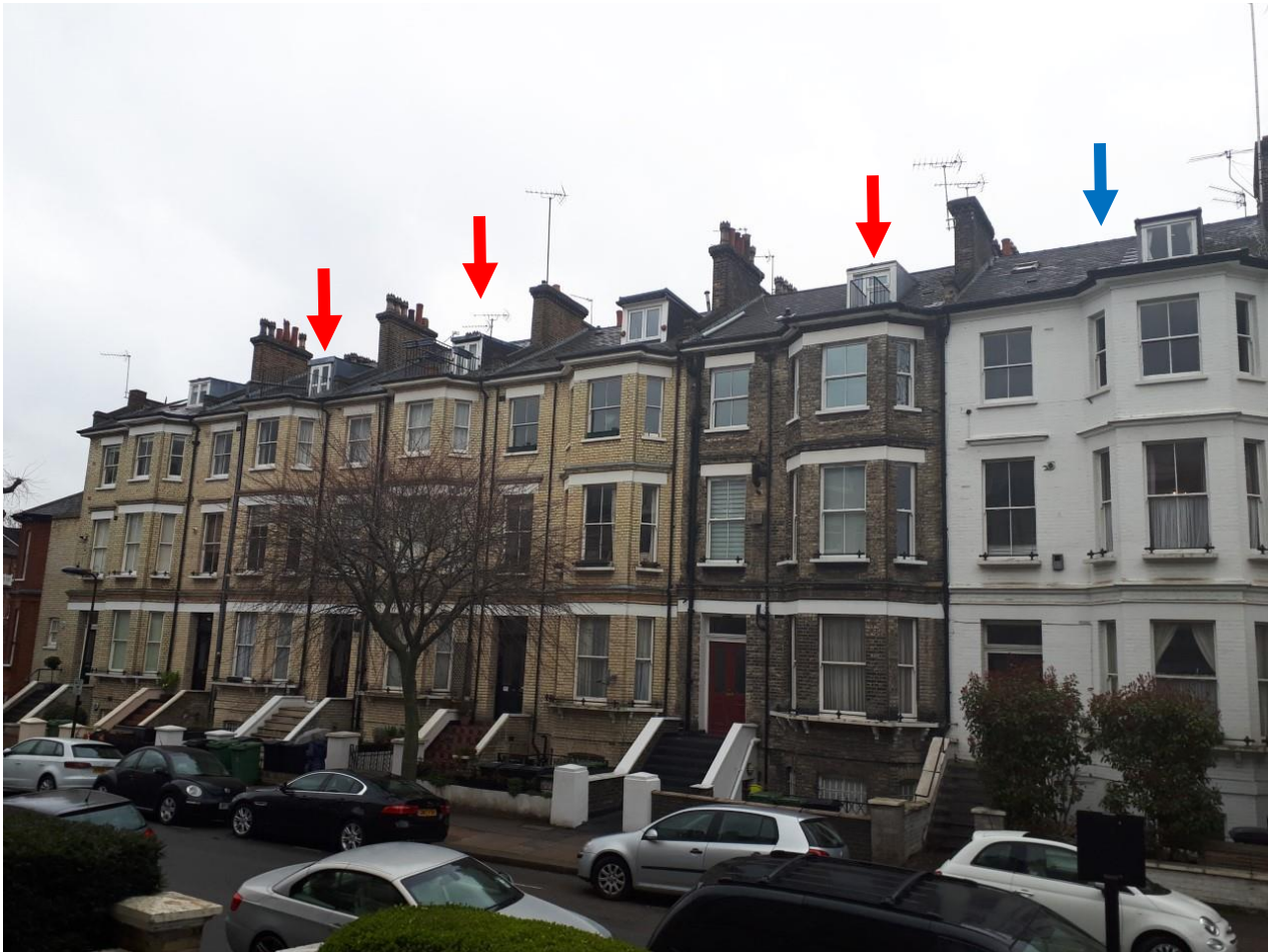
Plate 4. View from street level showing the 3no. existing front balconies and associated railings within the wider street (demarcated by red arrows). The appeal site is demarcated by a blue arrow.
