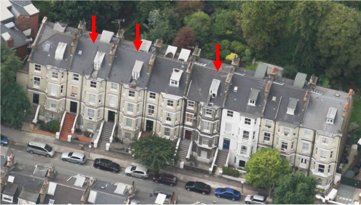
Plate 2. Properties on the west side of Crossfield Road showing the 3no. existing front balconies.
