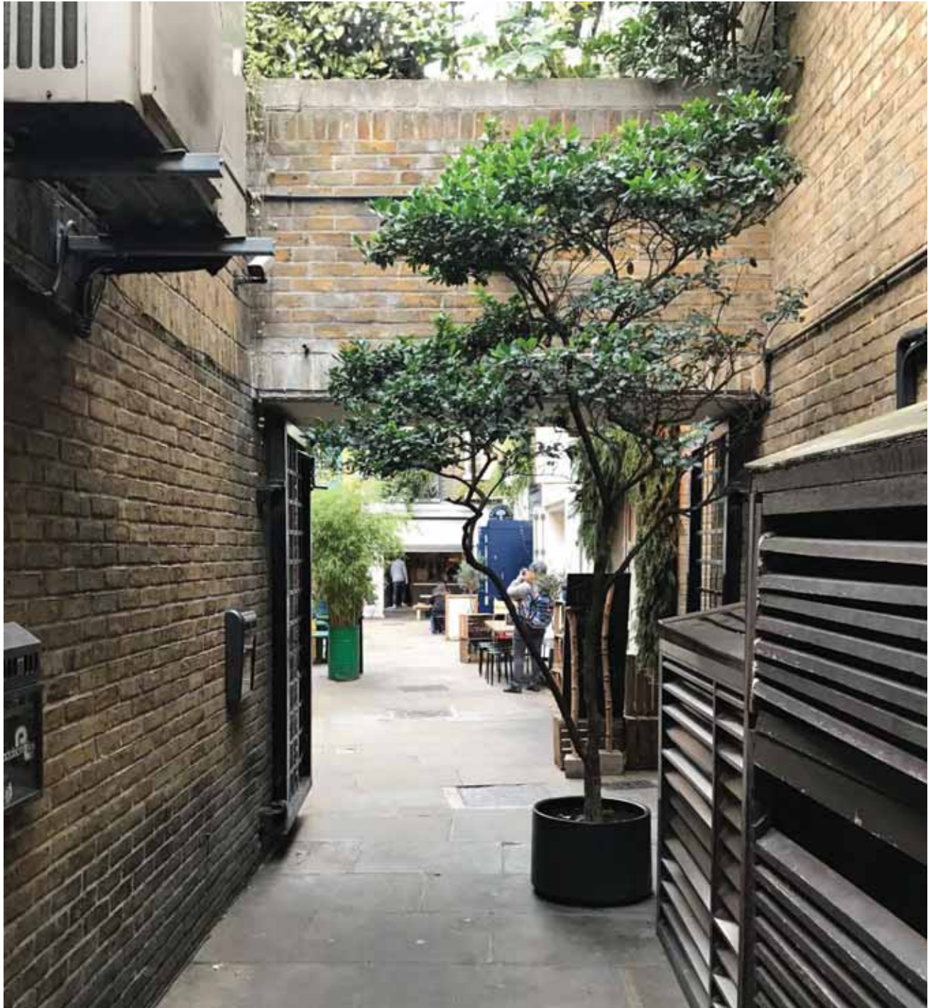
The proposed location of the condenser unit is in the wall to the left in this image, which also shows the existing enclosed condensers at ground level
