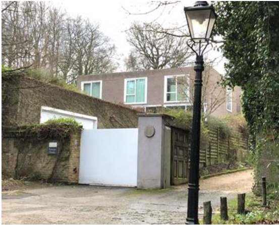
Figure 1: Image of Terrace House from North End Avenue
