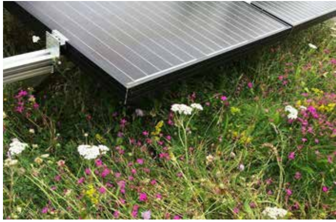
Solar PV and integrated green roof
