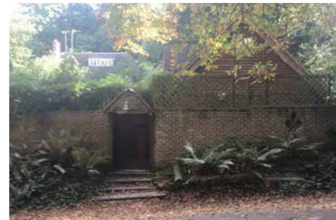
Street view of boundary wall and entrance to the site
