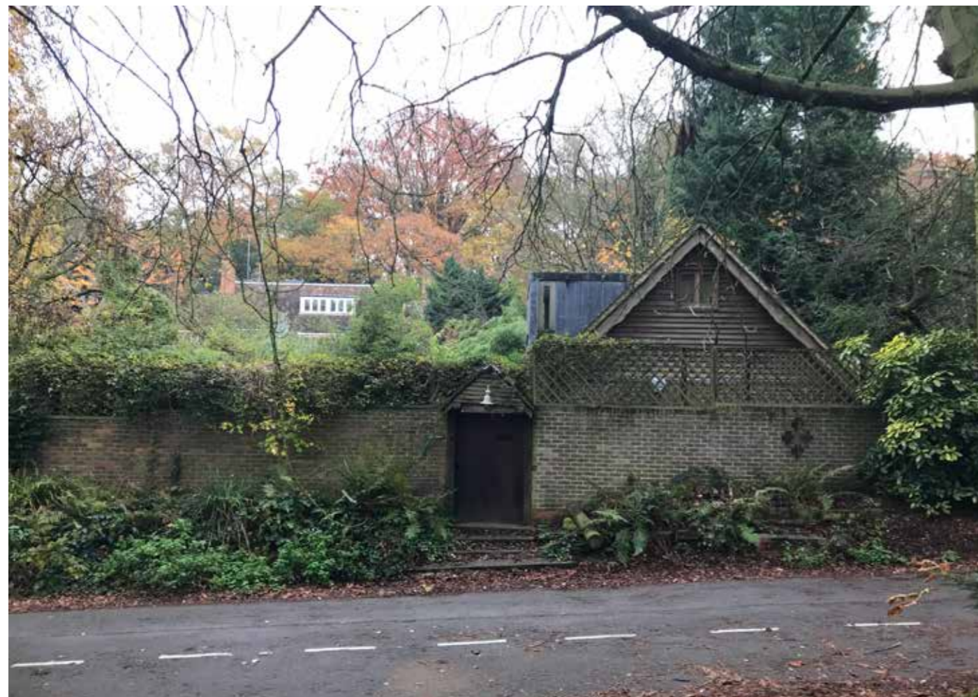
Photograph of Existing West Elevation
