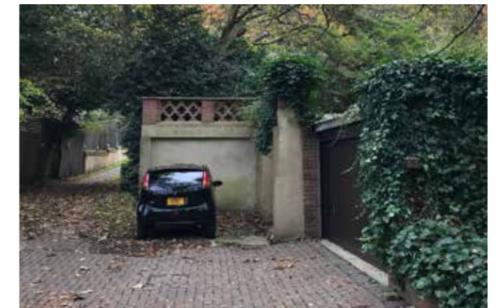
Modern garage brick wall and driveway to the northern boundary
