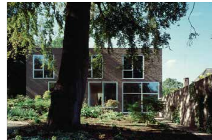
Terrace House, North End Avenue
