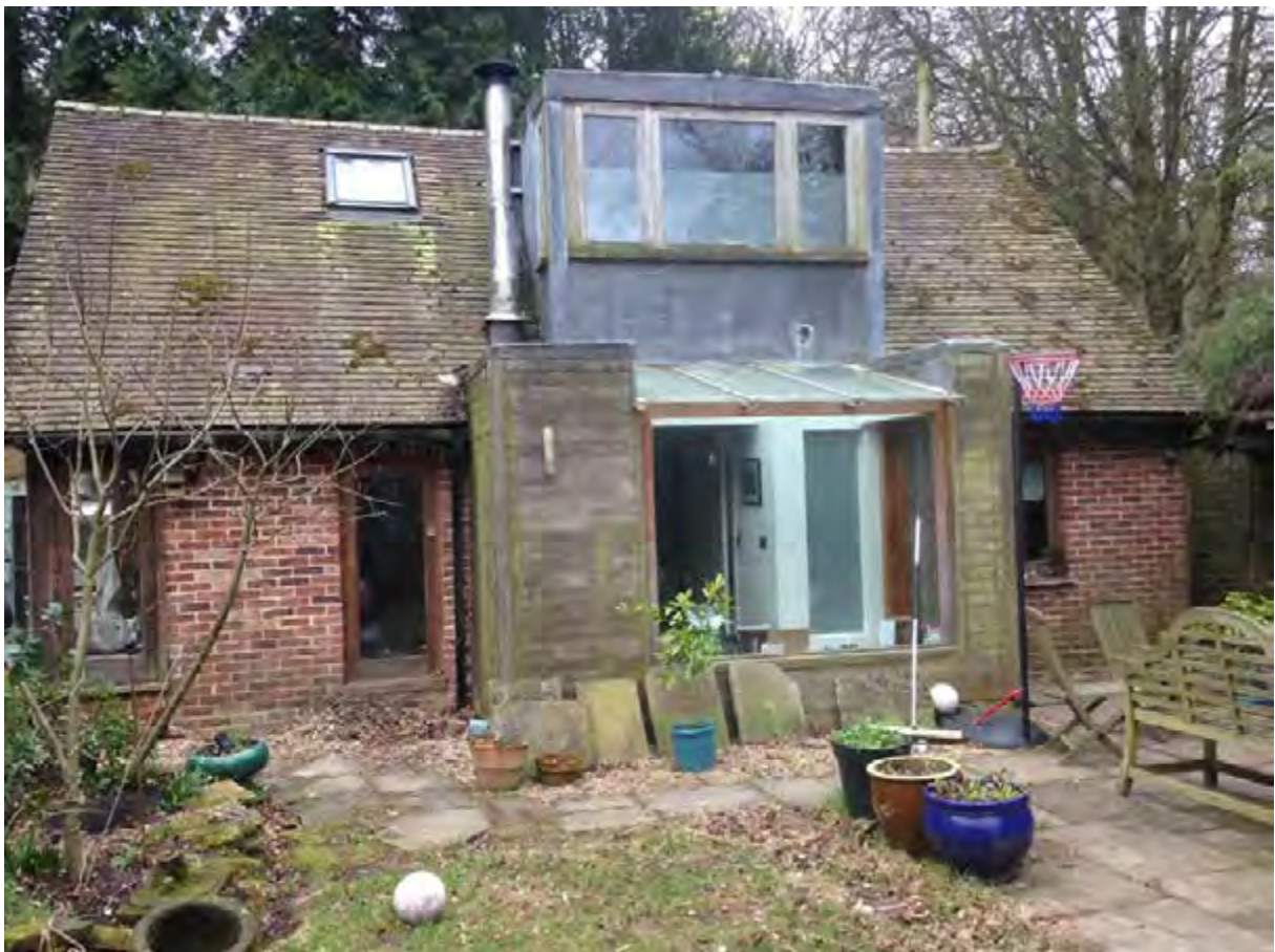
Plate 2: View facing south of The Studio residential property
