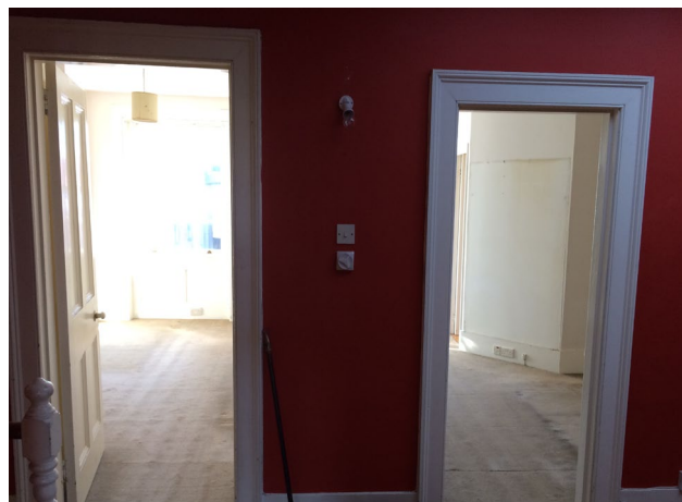
Existing doors to Bedroom 1 and 2
