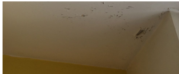
Bedroom 1 Ensuite - Ceiling
