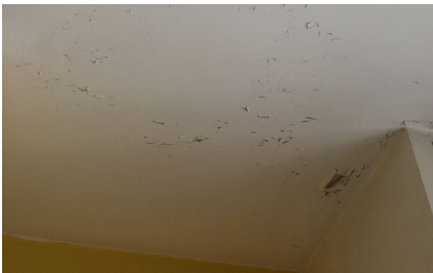
Bedroom 1 En-suite - Ceiling
