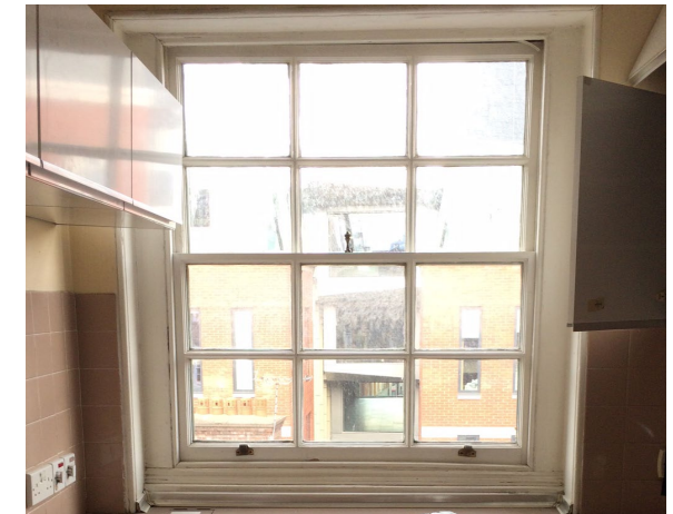
Existing Kitchen Window - Cill to be lowered
