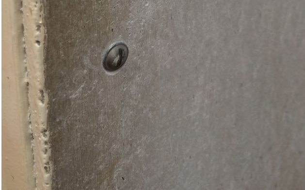
Asbestos Lining
