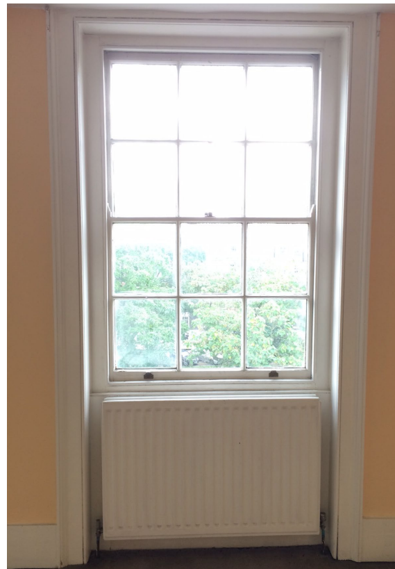
Existing Reception - Window
