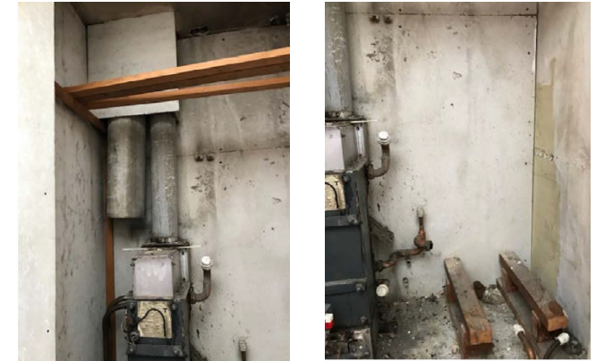
Removal of boiler and cylinder prior to asbestos removal.
