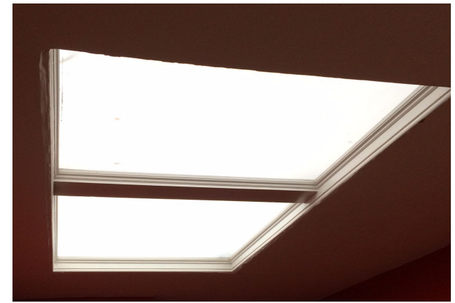
Hall - Immediately outside kitchen
