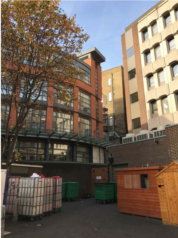
Photograph 3: Holborn Town Hall adjacent to service yard
