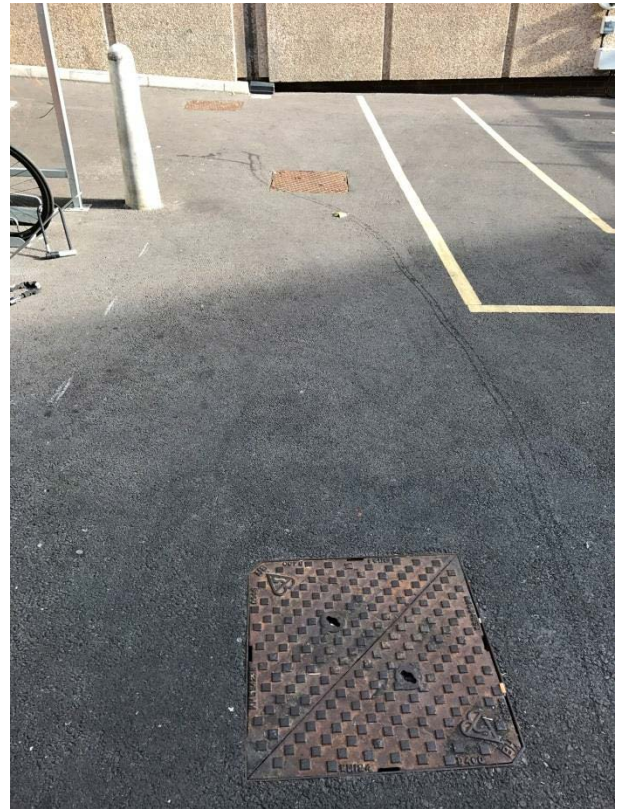
Photograph 7: Manholes within service yard
