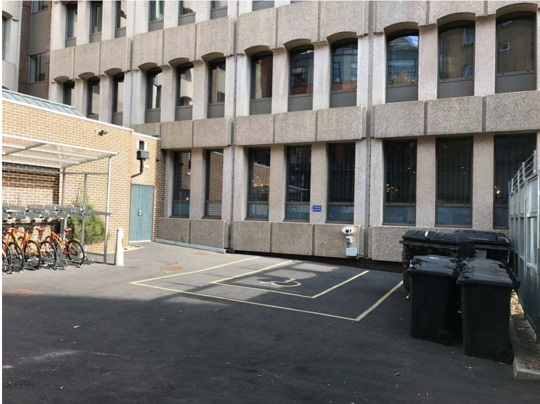
Photograph 1: Hoxton Hotel service yard looking east
