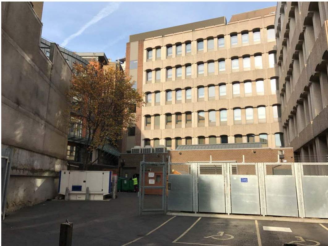
Photograph 2: Hoxton Hotel service yard looking north
