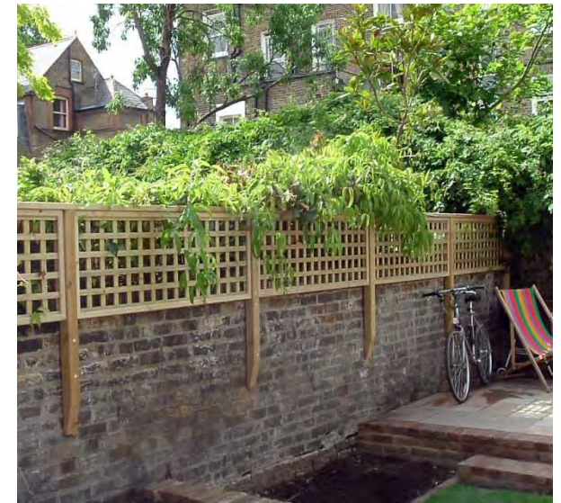
NORTH BOUNDARY FENCE TO BE REPLACED AND TOPPED WITH SMALL TRELLIS AS PER IMAGE ABOVE.
