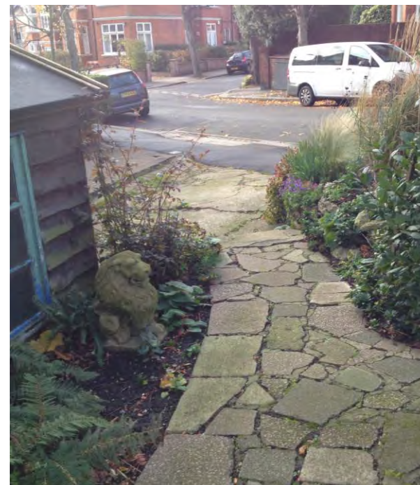
EXITING CONCRETE PATHS.
