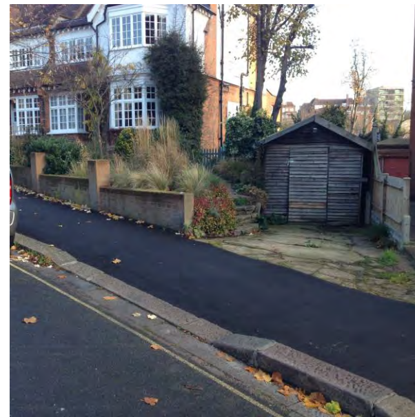
EXITING DRIVE, DROP KERB AND FRONT WALL. SMALL SECTION OF WALL WOULD BE REMOVED TO MAKE DRIVE WIDER.
