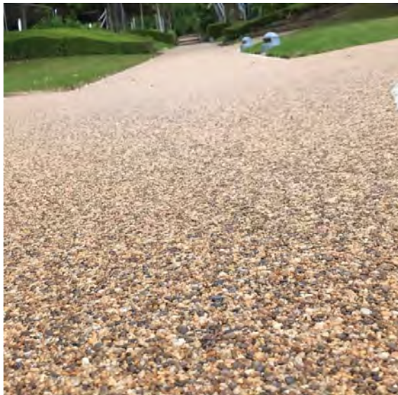
BARLEY BEACH PERMEABLE RESIN BOUND GRAVEL DRIVEWAY
