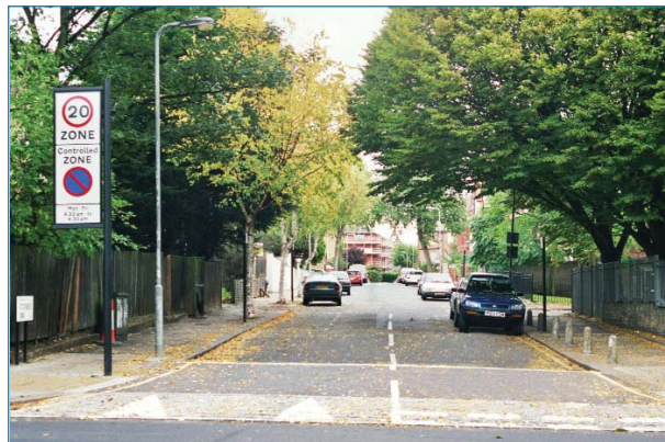
Raised entry treatment in St Cuthberts Road
