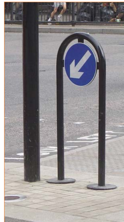
Externally illuminated metal hoop ‘keep left’ sign
