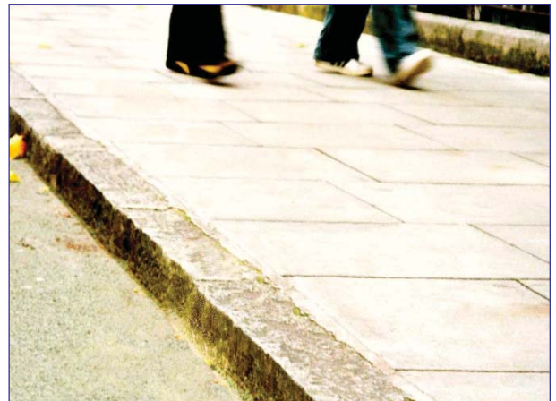
Boulevard paving laid with 150mm staggered bond
