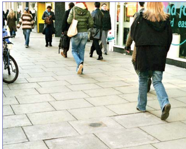
Boulevard paving on a busy commercial street
