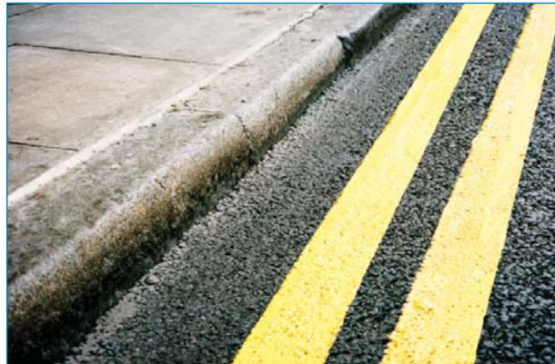
Canary yellow lines at 100mm width
