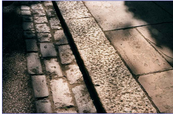
Flat kerb with drainage channel made of granite setts
