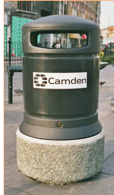
Heavy duty bin with concrete anchor
