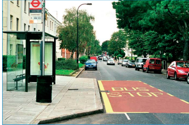
Bus boarder in Belsize Road
