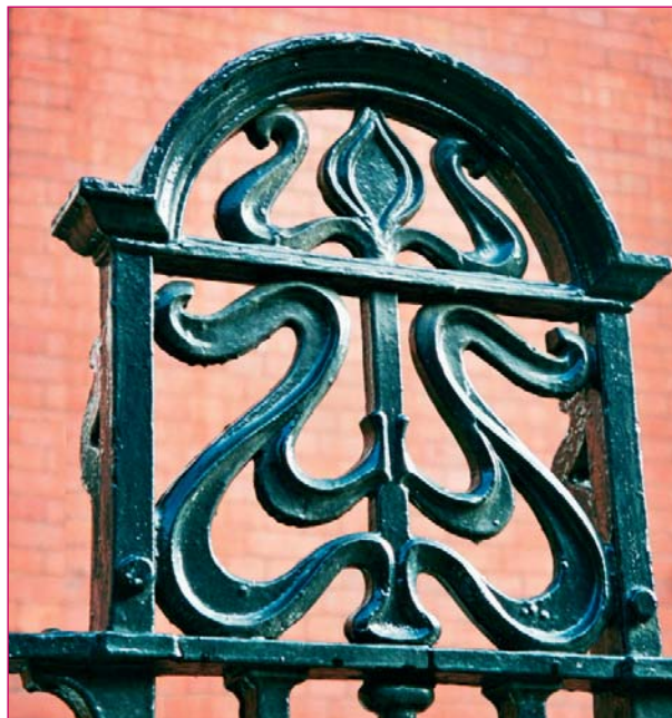
Railings in Bidborough Street
