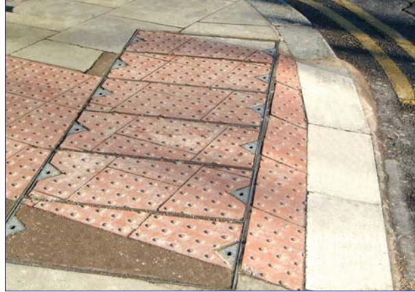
Continuity of tactile paving maintained through inset inspection cover
