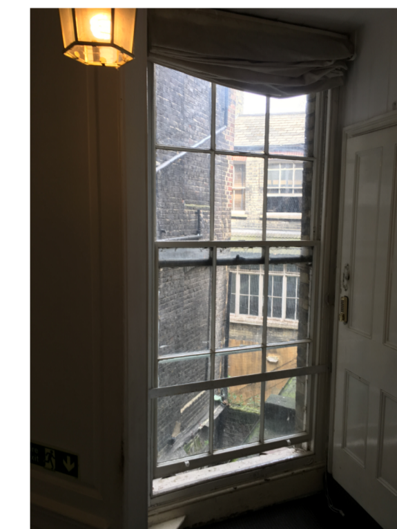
EXISTING WINDOW W.1.8
