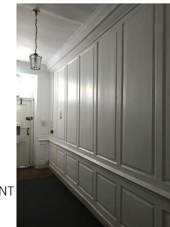
TIMBER PANEL SEEN FROM COMMON HALLWAY.
