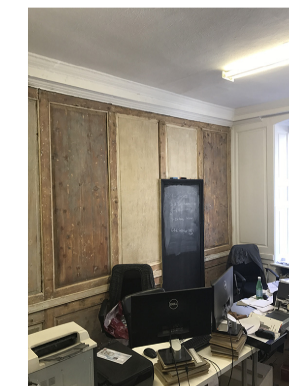
TIMBER PANEL SEEN FROM OFFICE.
