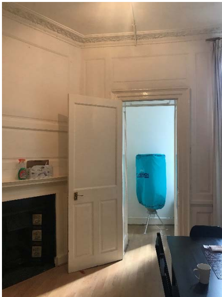
Fig 10 First floor door DR.1.5 and Lath & Plaster ceiling with cornice
