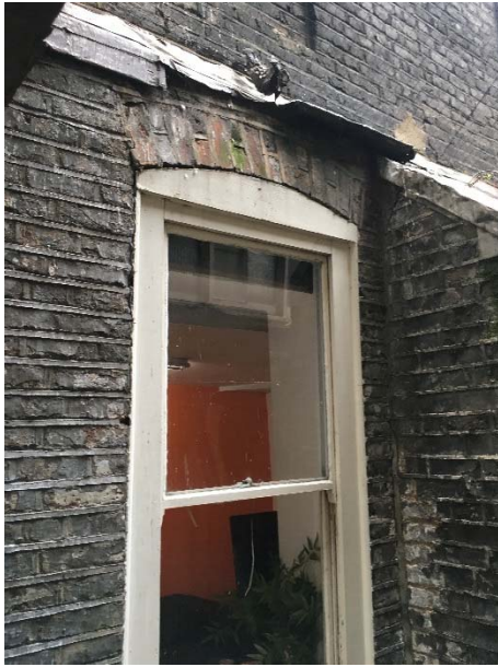
Fig 11 Rear basement light well window W.B.5 showing deformed lintel
