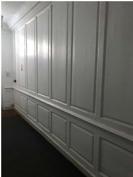
Fig 4 Ground Floor common hallway RM.0.1 timber panel wall
