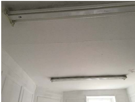
Fig 7 Ground floor ceiling without cornice seen in RM.0.4, plasterboard over lath & plaster
