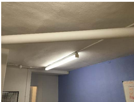
Fig 8 Basement floor ceiling without cornice seen in RM.B.5, plasterboard (unconfirmed lath & plaster above)
