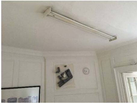
Fig 6 Ground floor ceiling with cornice seen in RM.0.3. Lath & Plaster.
