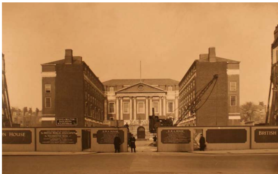
Early stages in the construction of Wontner Smith's extensions for BMA House in 1929.
