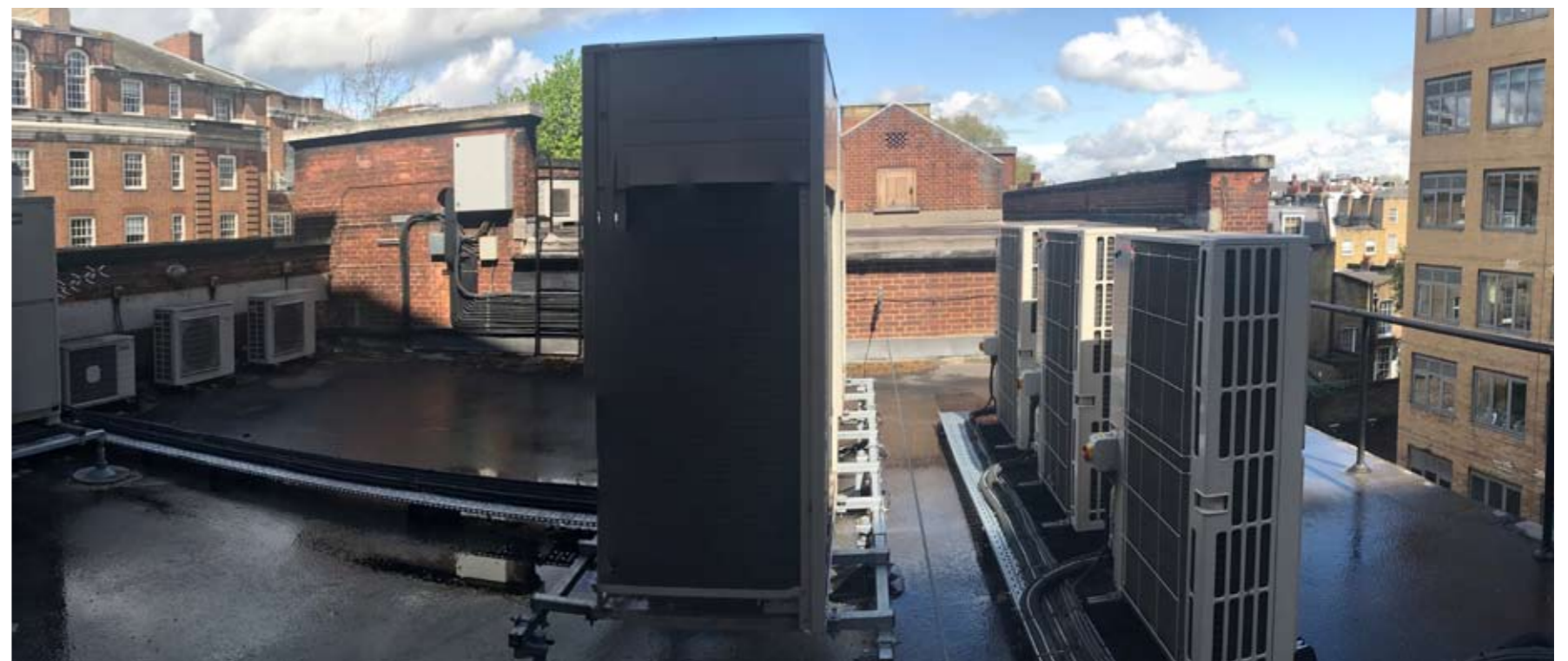
Panoramic views of the existing rooftop area.
