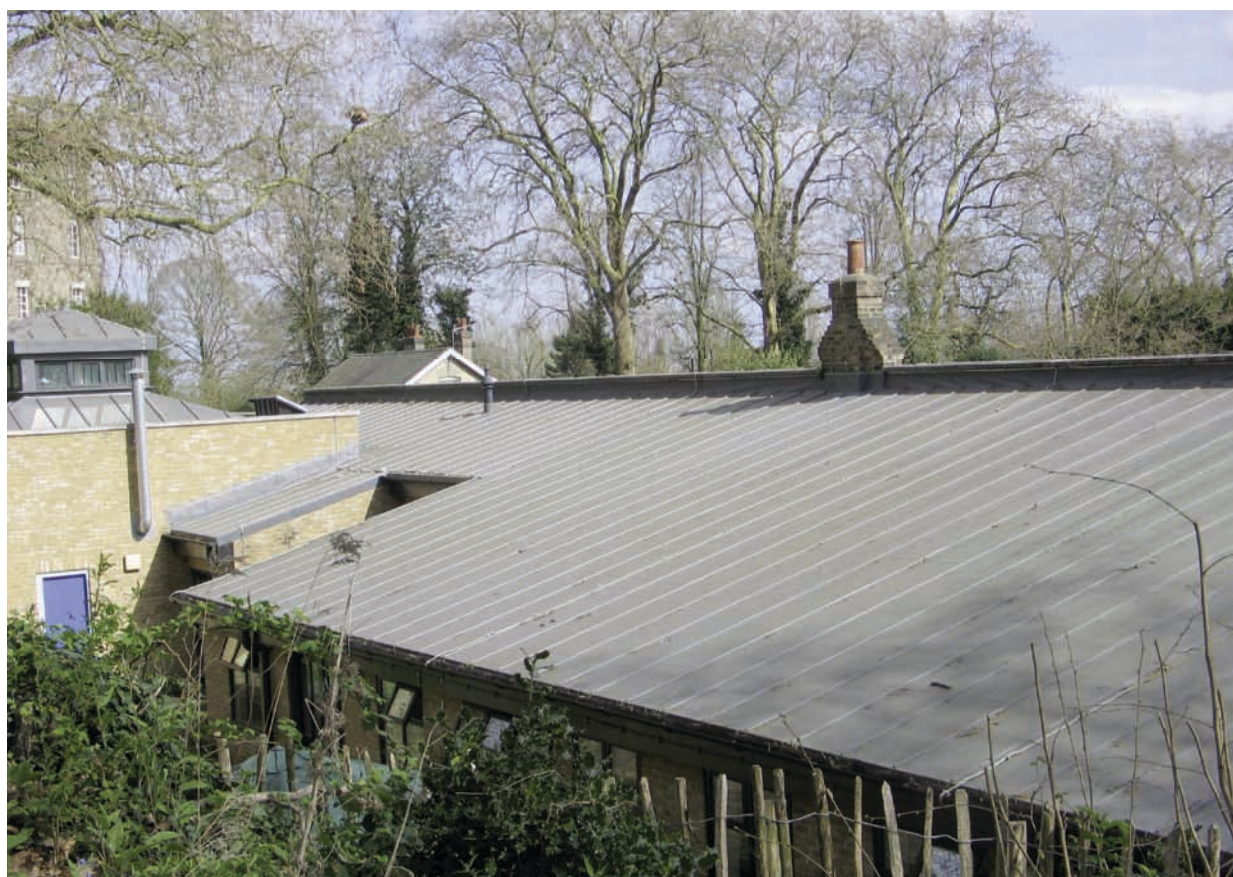
Pitched roof to rear, with Sarnafil single ply membrane
