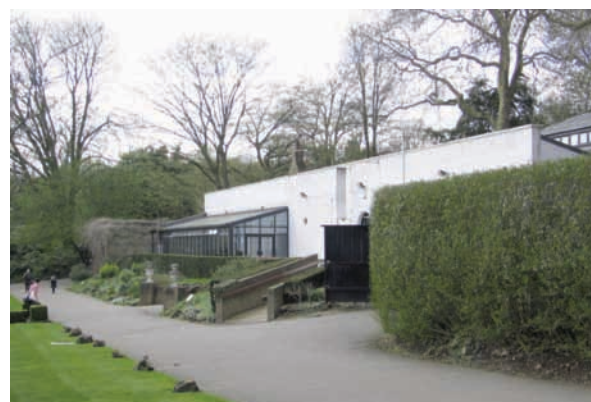
2- View of entrance from east
