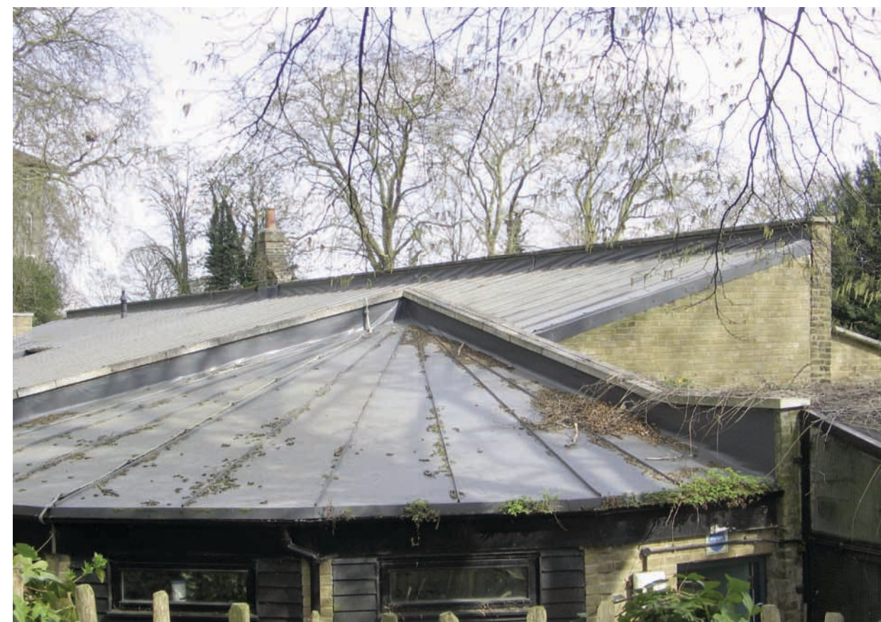
Pitched roof to curved area at west end of building
