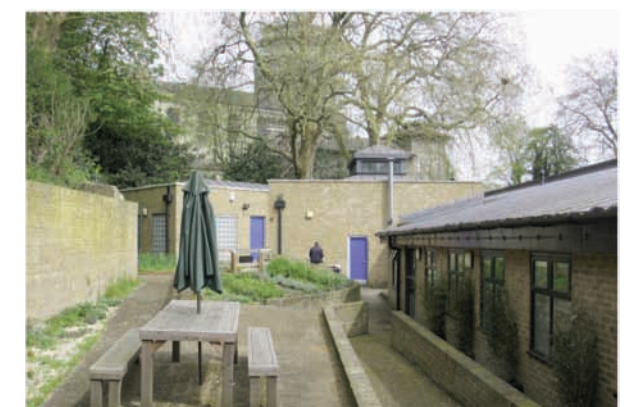
Retaining wall and change in level
