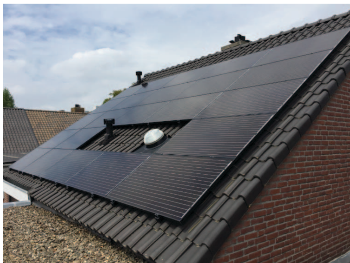
All black monocrystalline silicon pv panels installed
