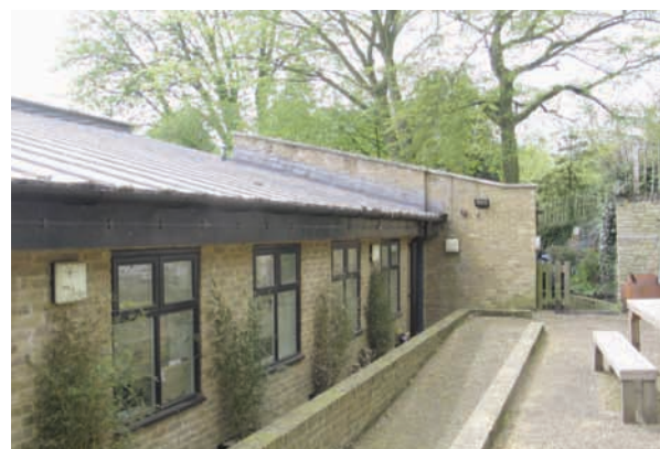
7- rear courtyard looking west
