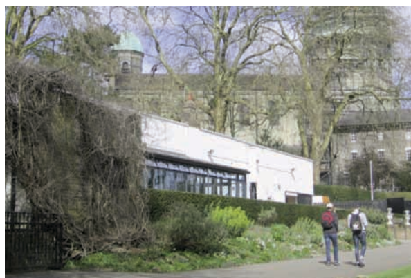
1- View of entrance from west
