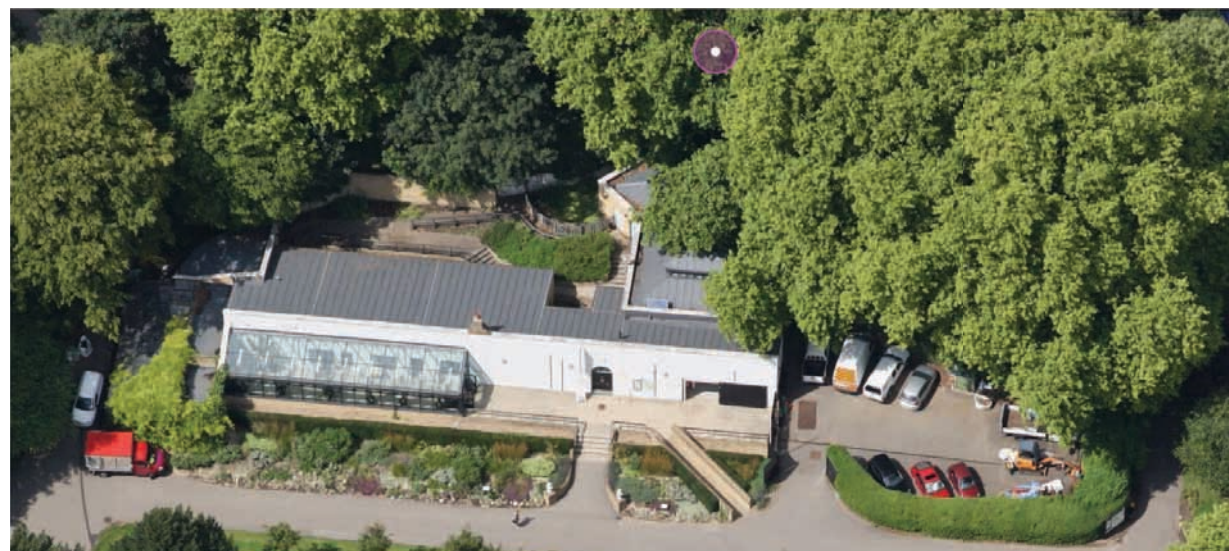
Waterlow Park Centre, showing retaining wall and planting to the north of the building
