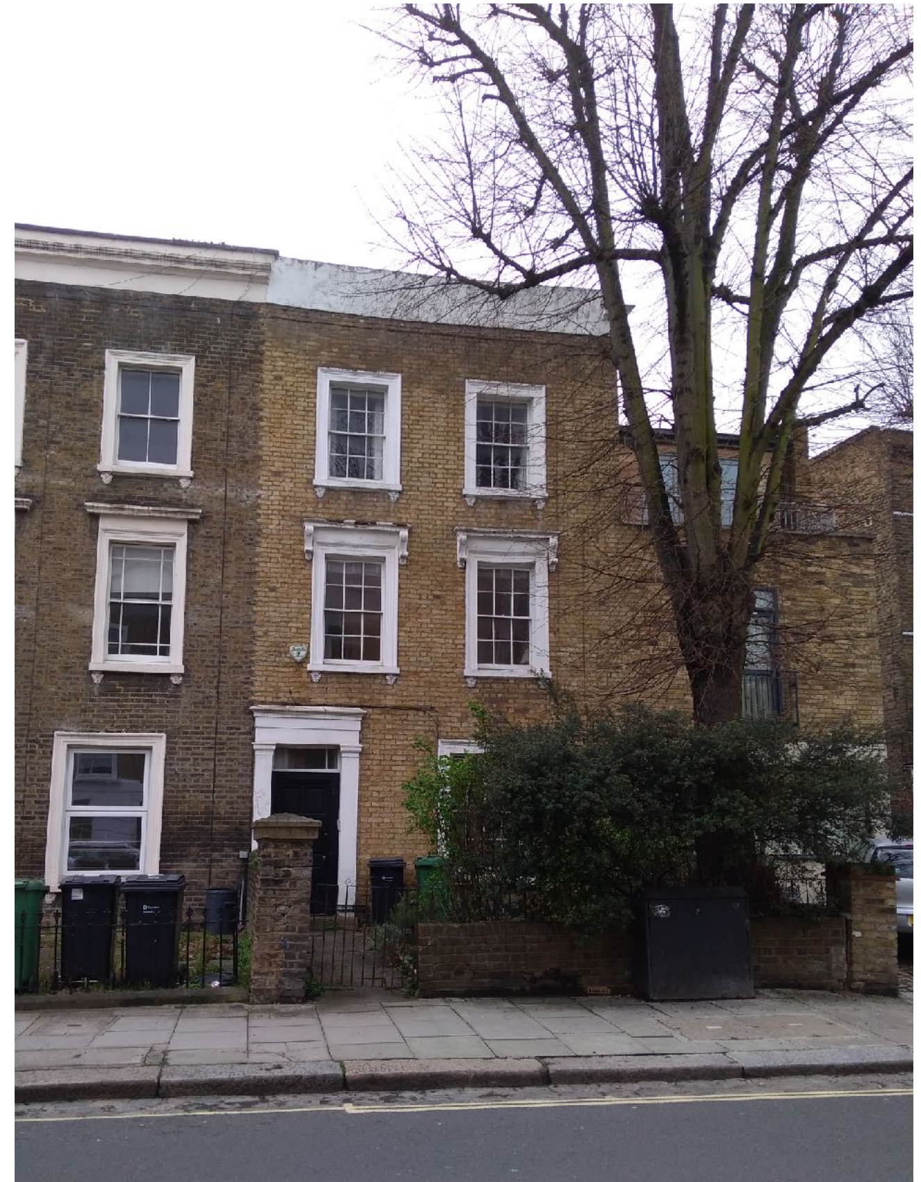
Front street elevation of 31 Grafton Road
